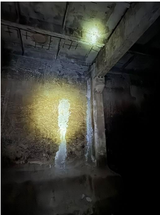
Photo 3-9 Damaged waterproofing layer of the water reservoir No. 2
