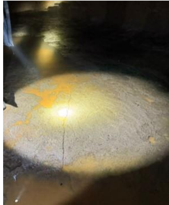
Photo 3-3 Crack on the bottom of the water reservoir No. 1
