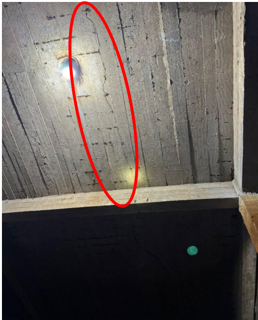
Photo 3-4 Crack on the beam of the water reservoir No. 1
