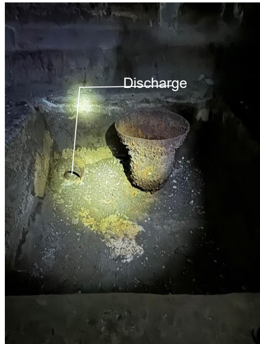
Photo 3-10 Damaged drain pipe of the water reservoir No. 2
