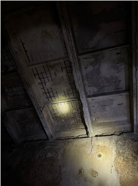
Photo 3-7 Damaged roofing tile of water reservoir No. 2
