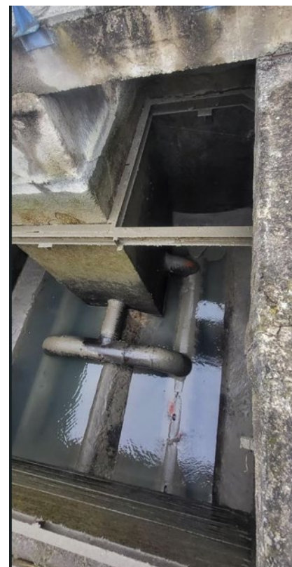
Existing settlement tank inlet zone– Distribution chamber
