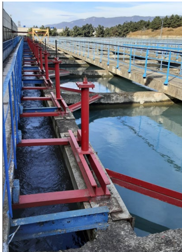
Existing settlement tanks– Outlet channel to filtration stage
