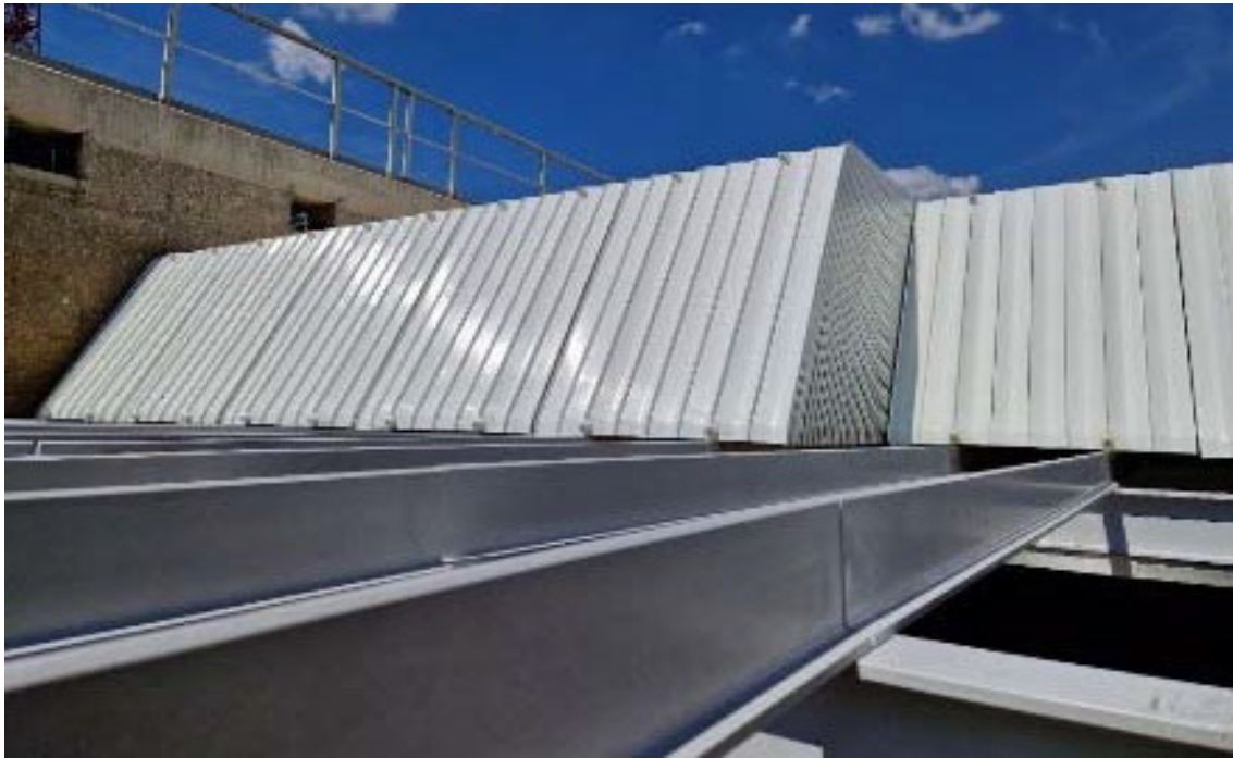
Lower view of new lamella modules and supports
