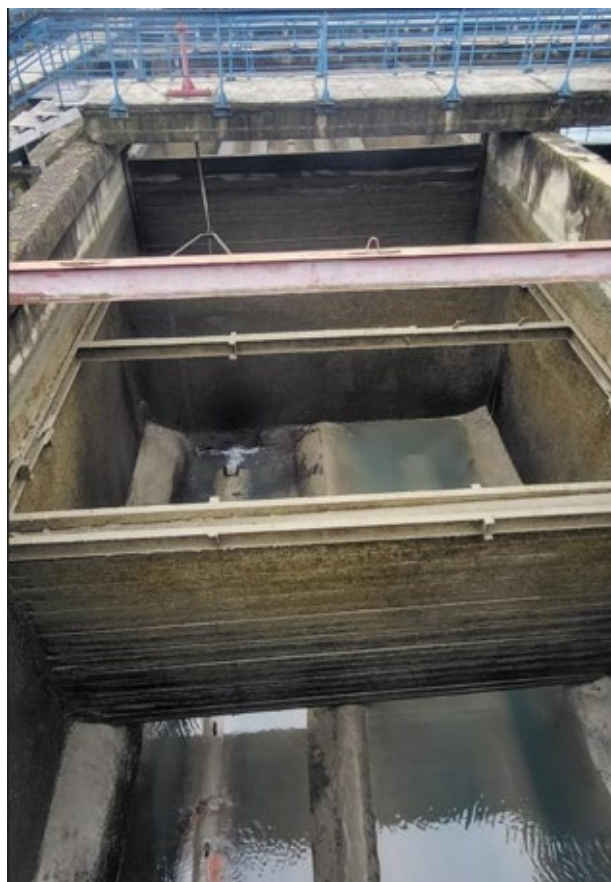
Existing settlement tank flocculation zones & Stream baffles – View from distribution chamber
