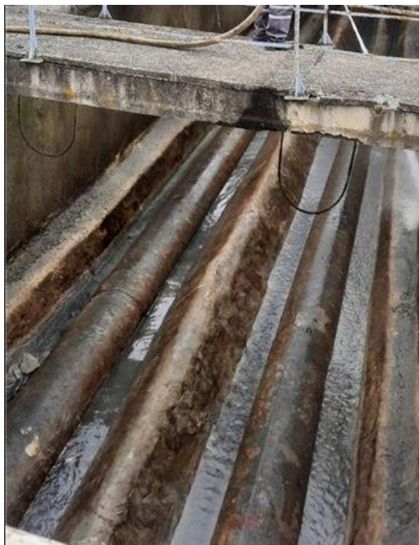
Existing settlement tank static zones & sludge draw-off piping
