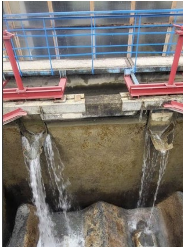
Existing settlement tank– Outlet penstocks to filtration stage feeding channel
