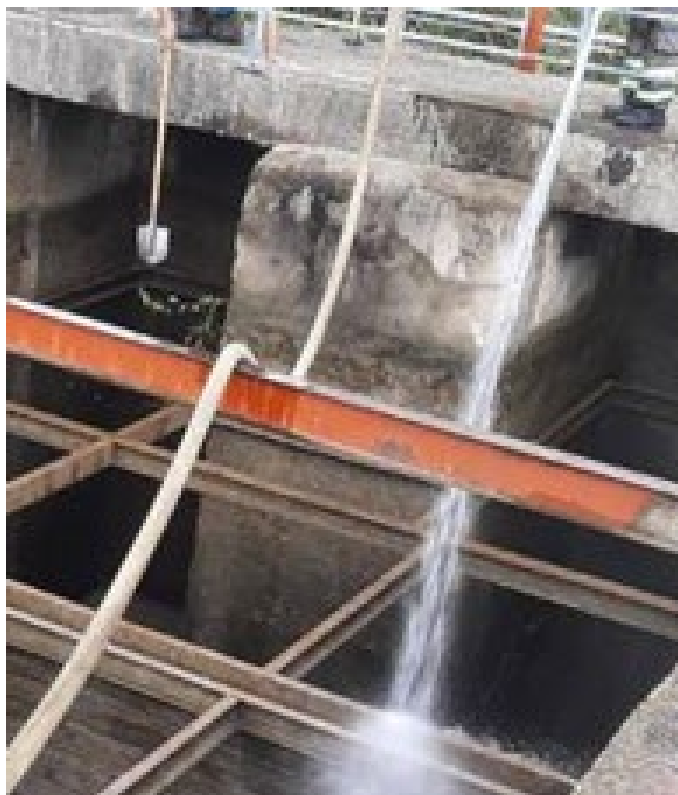
Existing settlement tank inlet zone– Distribution chamber
