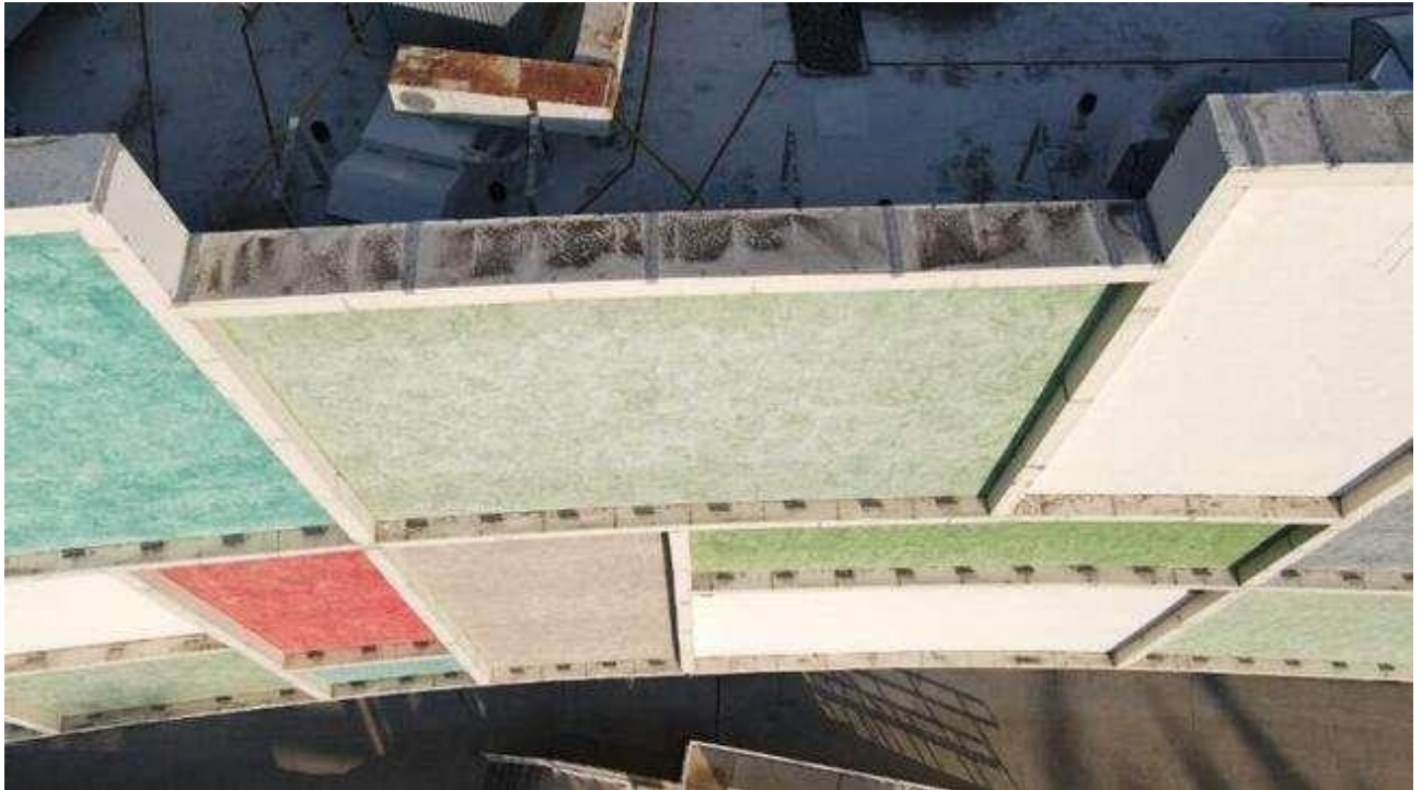
Figure 5.1.10. Drip molding along the upper edge of the facade. The joints of the drip molding are treated with sealant
