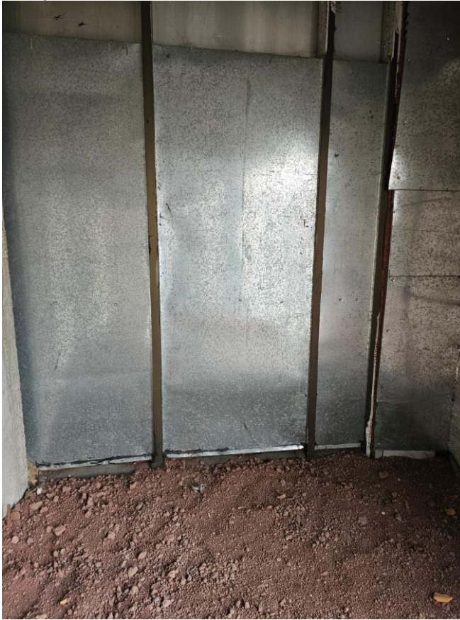
Figure 5.2.27. The ventilation grilles are currently not functional. These grilles are subject to leaks from precipitation (indirect defects). The inside is sealed with steel sheets and polyurethane sealant.
