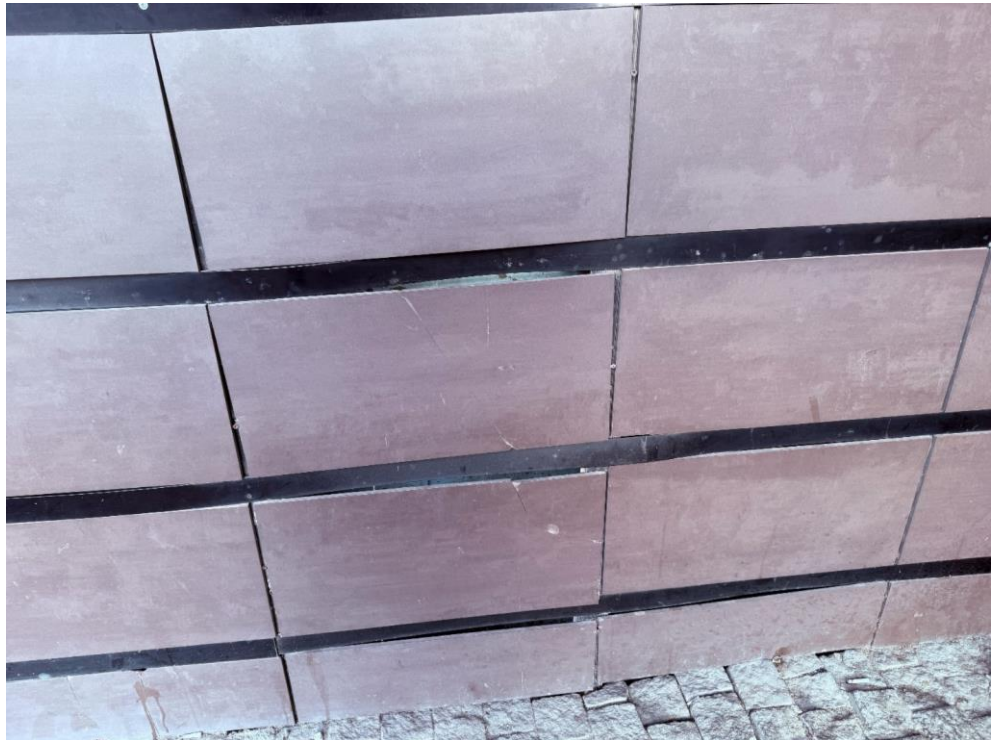
Figure 5.2.20. Delamination of battens and panels from the frame uprights. Cracks in the panels
