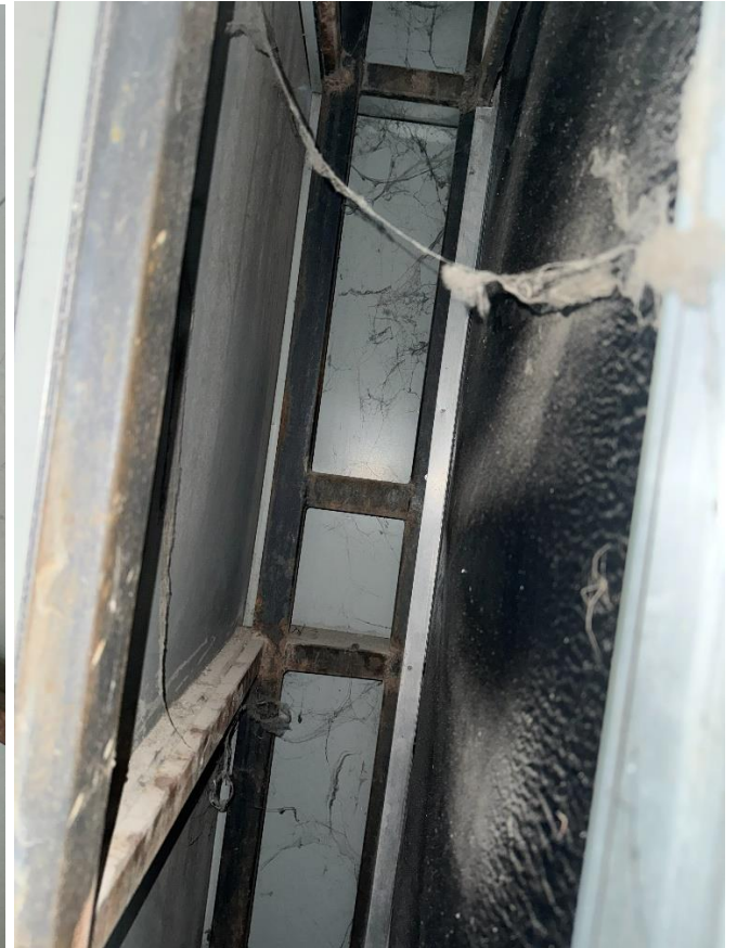
Figure 5.2.17. Corrosion of the frame of the suspended aluminum facade panels
