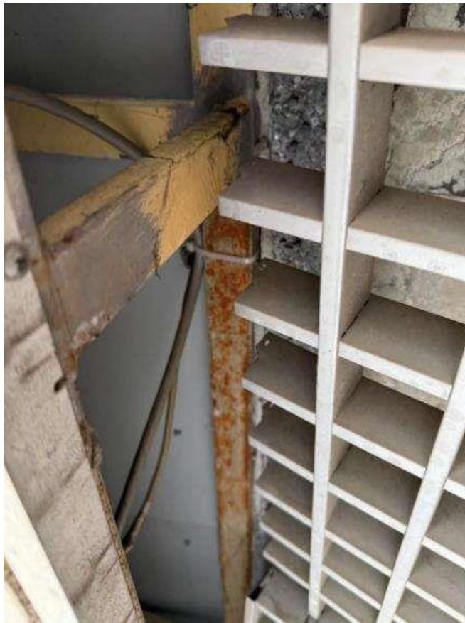
Figure 5.1.35. Fastening of the impost frame to the slab at elevation +6.000. Corrosion of frame elements. Lack of a support profile for the insulation. Non-continuous gluing of the insulation
