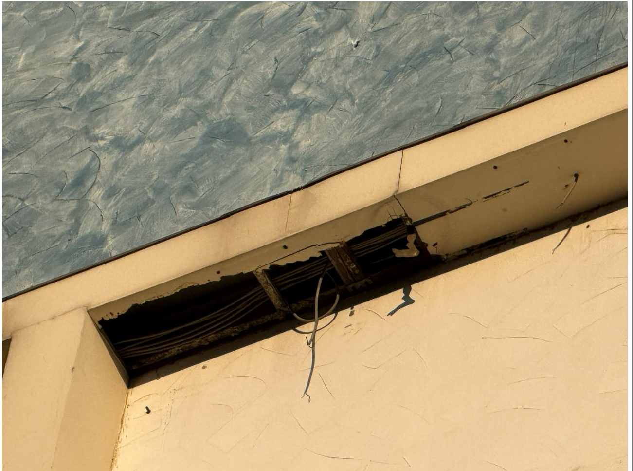
Figure 5.1.26. Destruction of the horizontal impost. Corrosion of the steel frame of the impost
