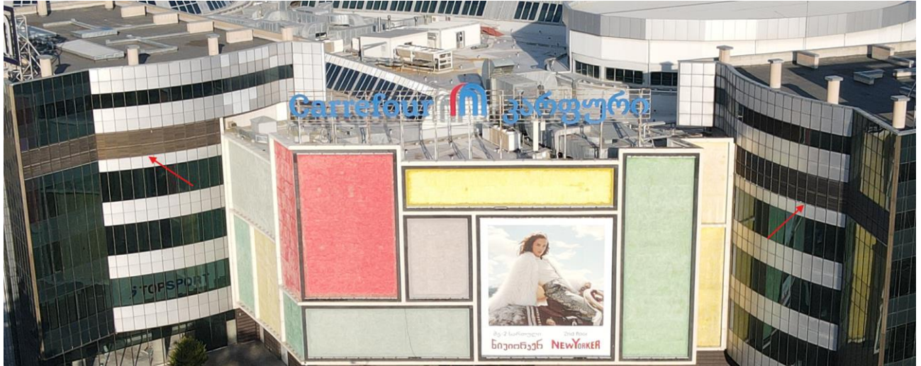
Figure 7.4. Ventilation grilles on the building facade
