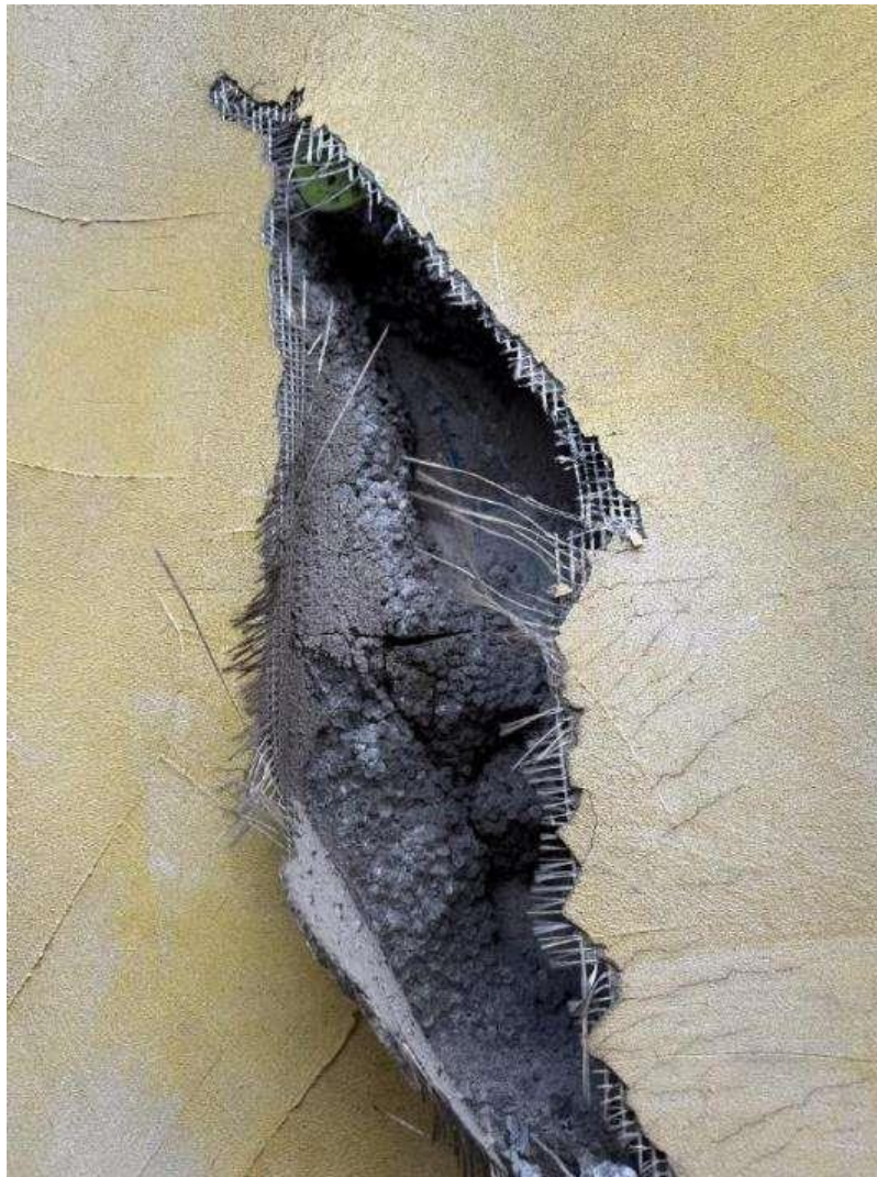
Figure 5.1.16. Localized damage to the PPS insulation layer
