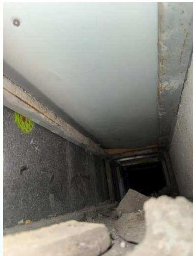
Figure 5.1.38. Opening of the horizontal impost. Areas of surface corrosion
