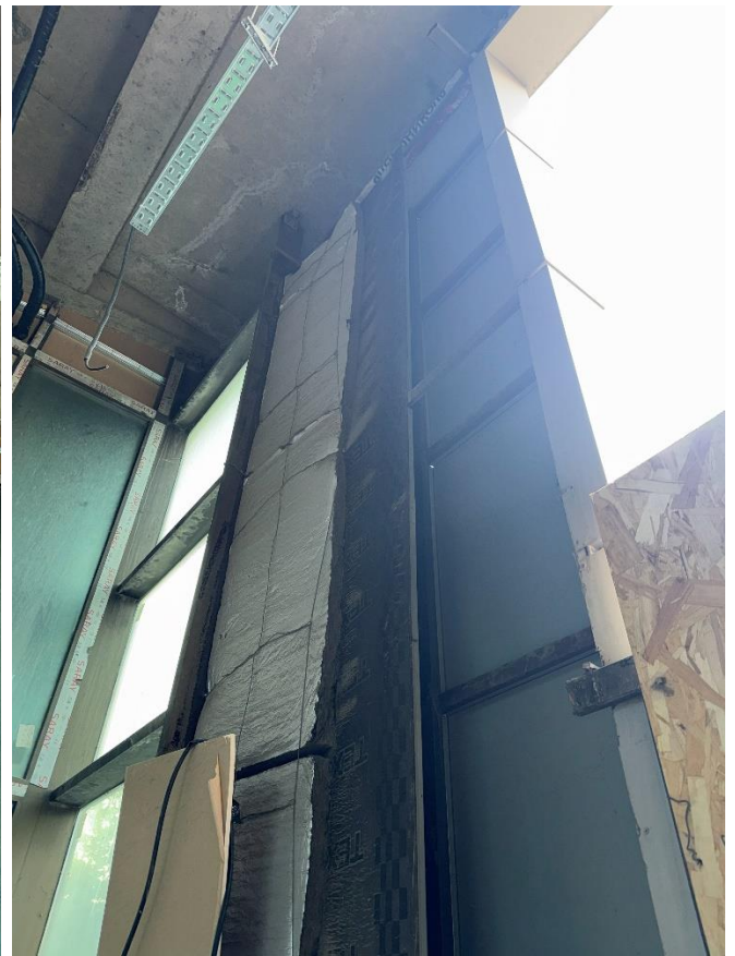
Figure 5.2.18. Insulation structure of this part of the facade
