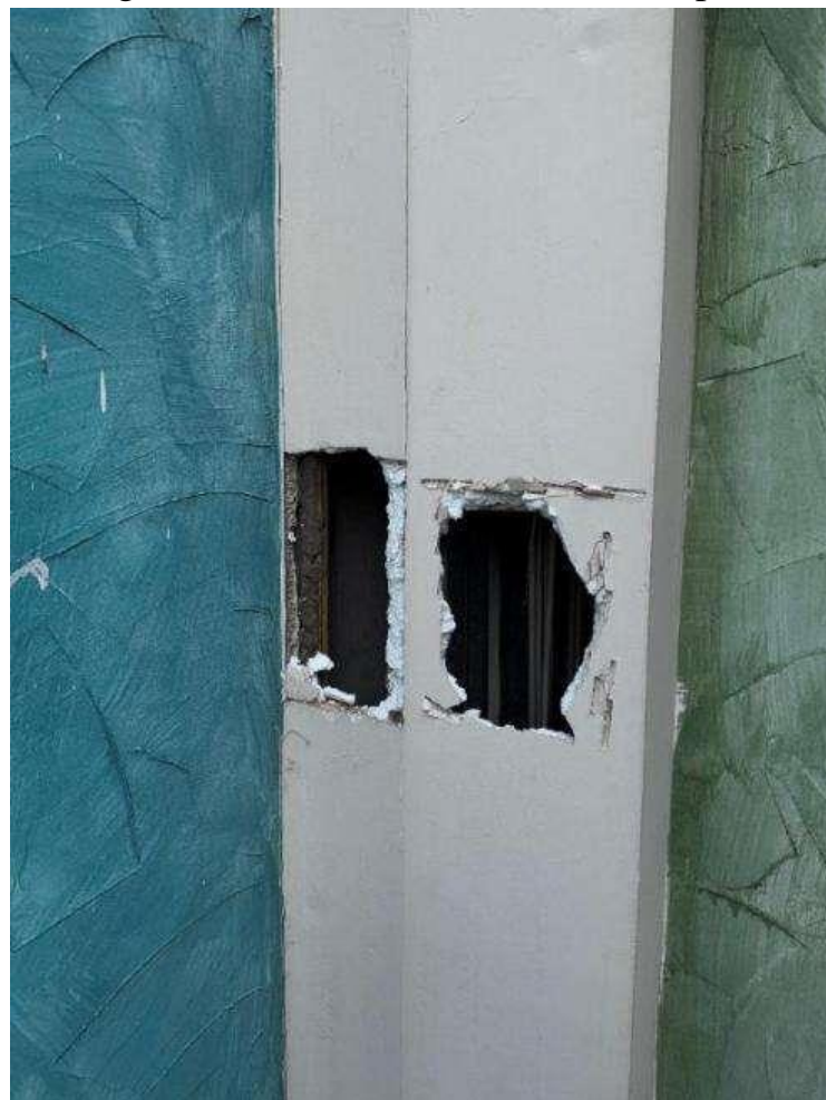
Figure 5.1.43. Opening the finishing layer of a vertical impost
