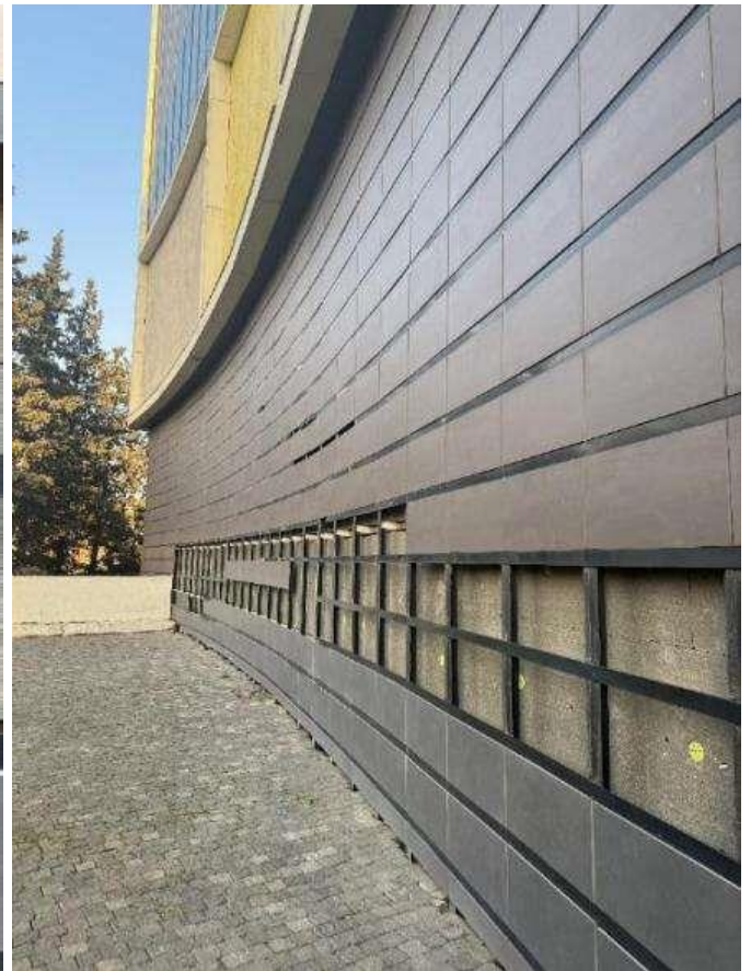
Figure 5.2.2. Fastenings of the insulation layer (insufficient). Increased gaps between slabs. Adhesive layer on the vertical fastening element of the ventilated facade
