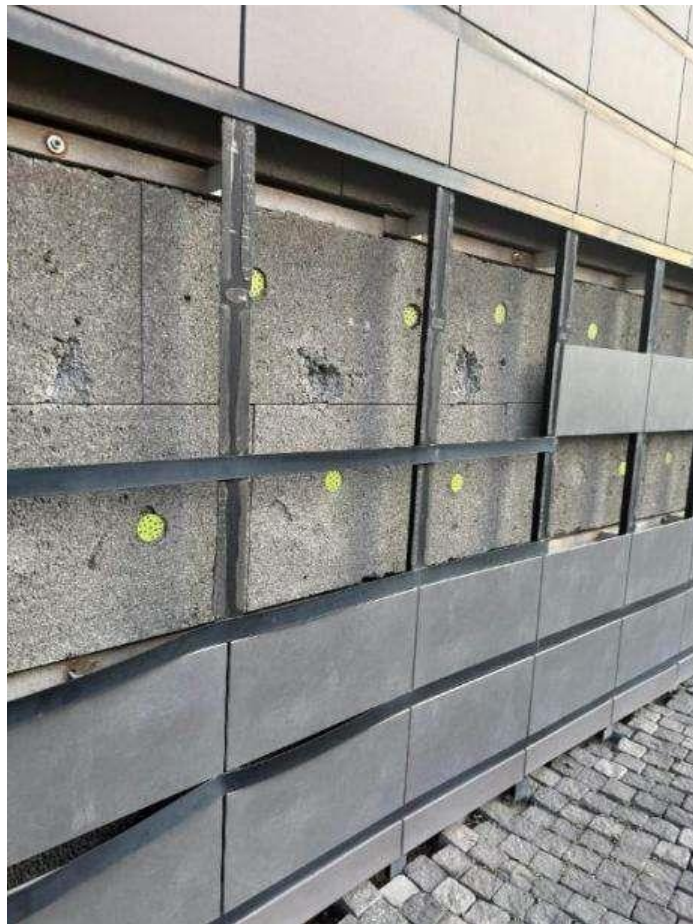
Figure 5.2.6. Detachment of slats and panels from frame posts
