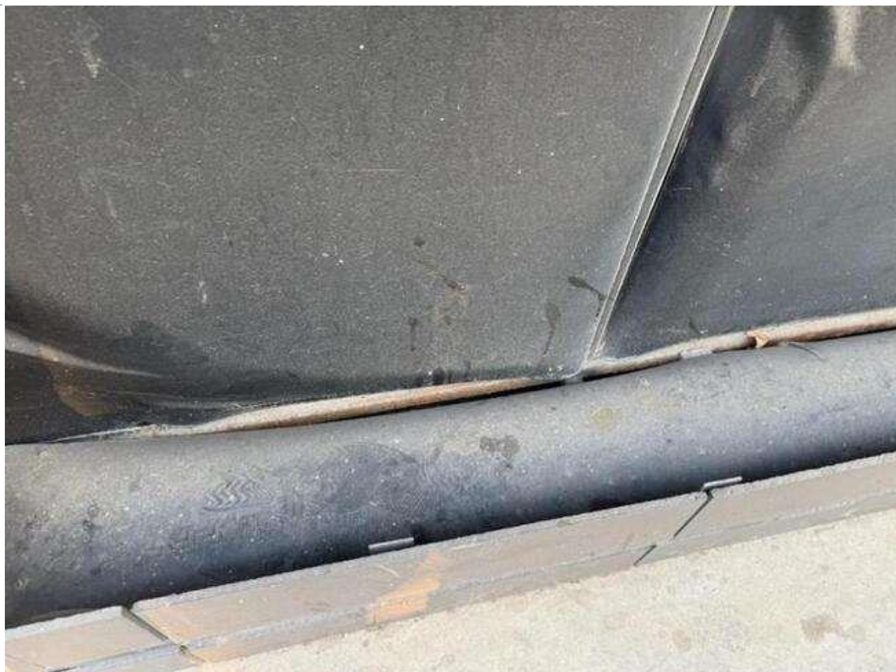
Figure 5.2.13. Destruction of the stitching in the inscription "TBILISI MALL" in axes 4-5/A. Corrosion of the facade system frame
