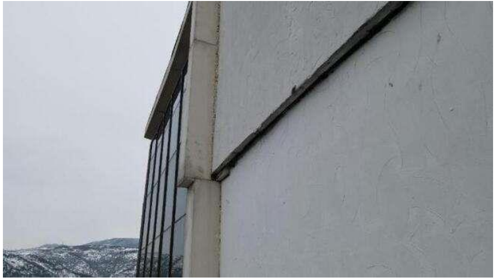
Figure 5.1.62. Crack on the facade of the building in axes 5-6/A. Delamination of the insulation layer.
