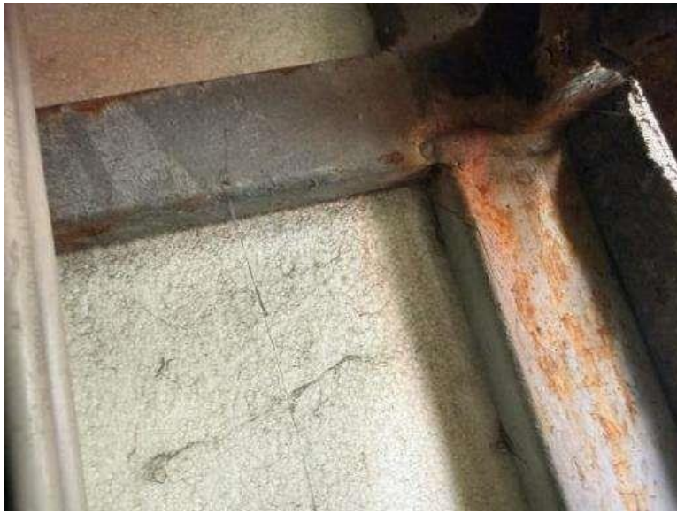
Figure 5.1.31. Connection of the vertical and horizontal frames of the facade impost. Surface corrosion
