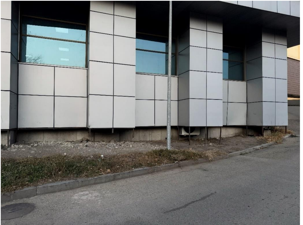
Figure 5.2.22. Facade construction made of suspended aluminum panels
