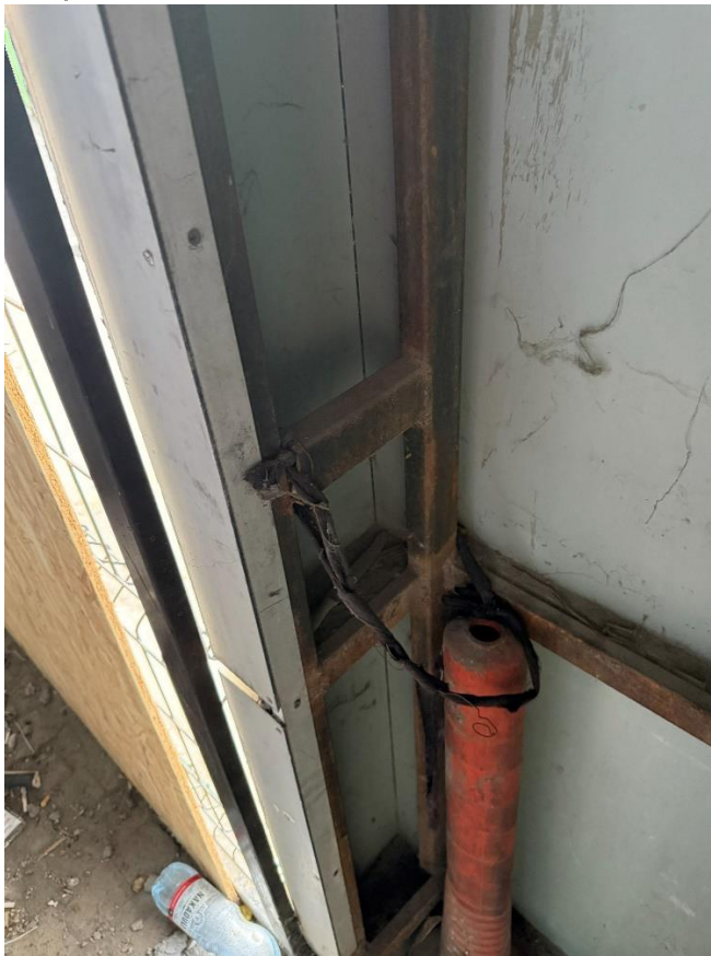
Figure 5.2.17. Corrosion of the frame of the suspended aluminum facade panels
