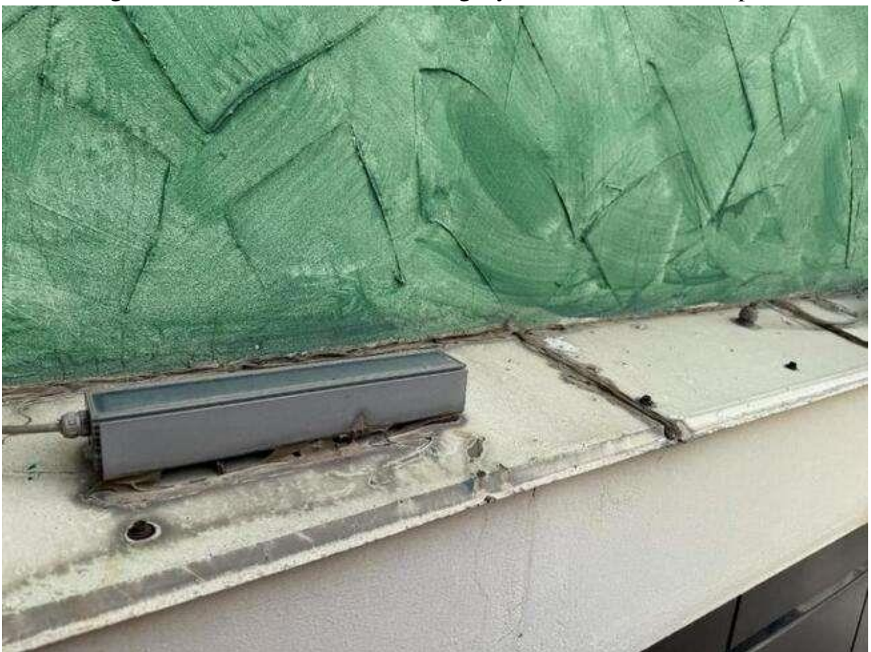
Figure 5.1.40. Sealant in the flashings of horizontal imposts
