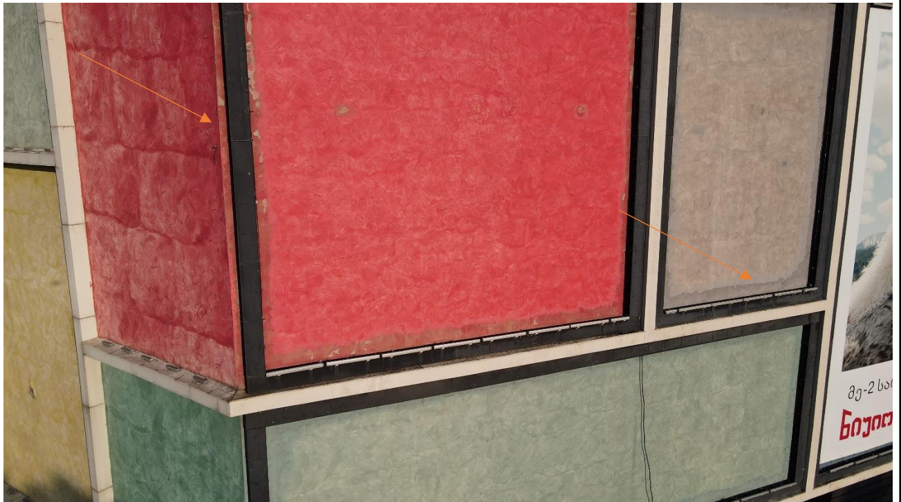
Figure 5.1.19. Space for a banner. Areas of facade damage
