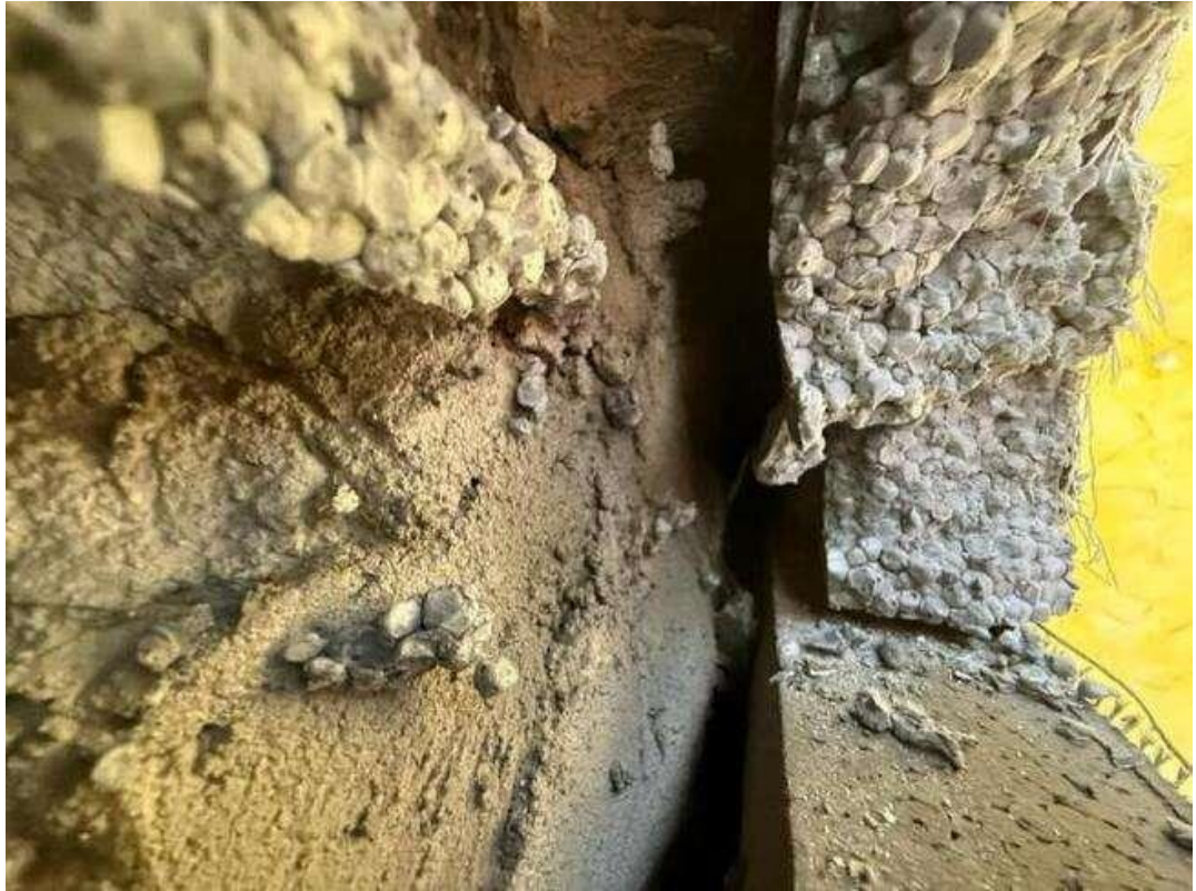
Figure 5.1.54. Gap up to 50 mm between the insulation and the wall
