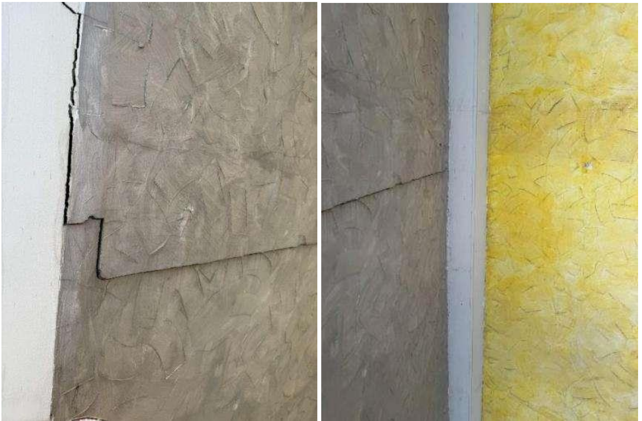
Figure 5.1.53. Crack on the facade of the building. Delamination of the insulation layer. This defect was caused by an uneven foundation and installation defects.
