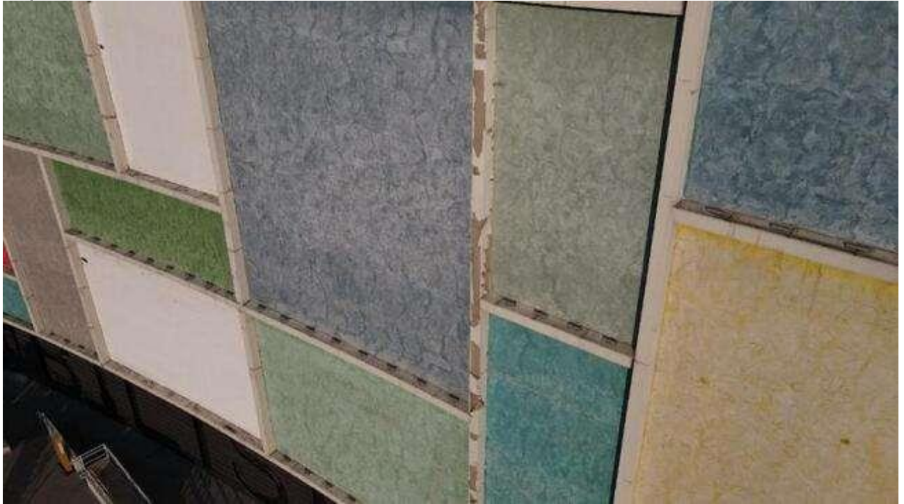
Figure 5.1.9. General view of the facade. Damage to the finishing layer of the impostes
