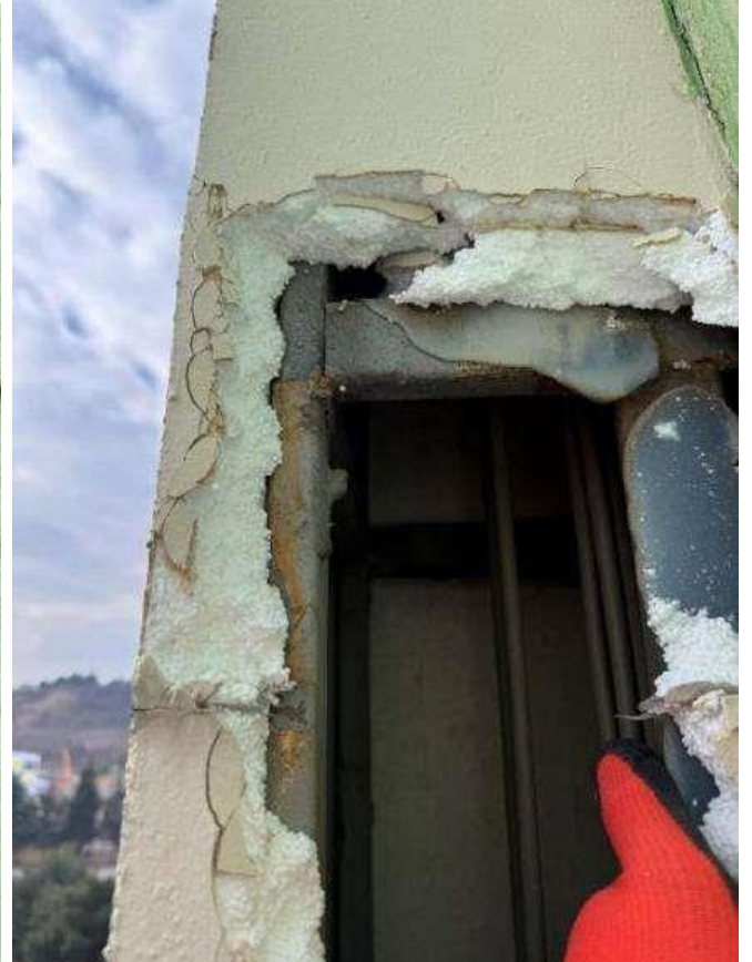
Figure 5.1.32. Opening of the vertical impost. Areas of adhesive bonding (non-continuous). This method of fastening is not standardized; similar solutions must also be mechanically fastened due to the small contact area
