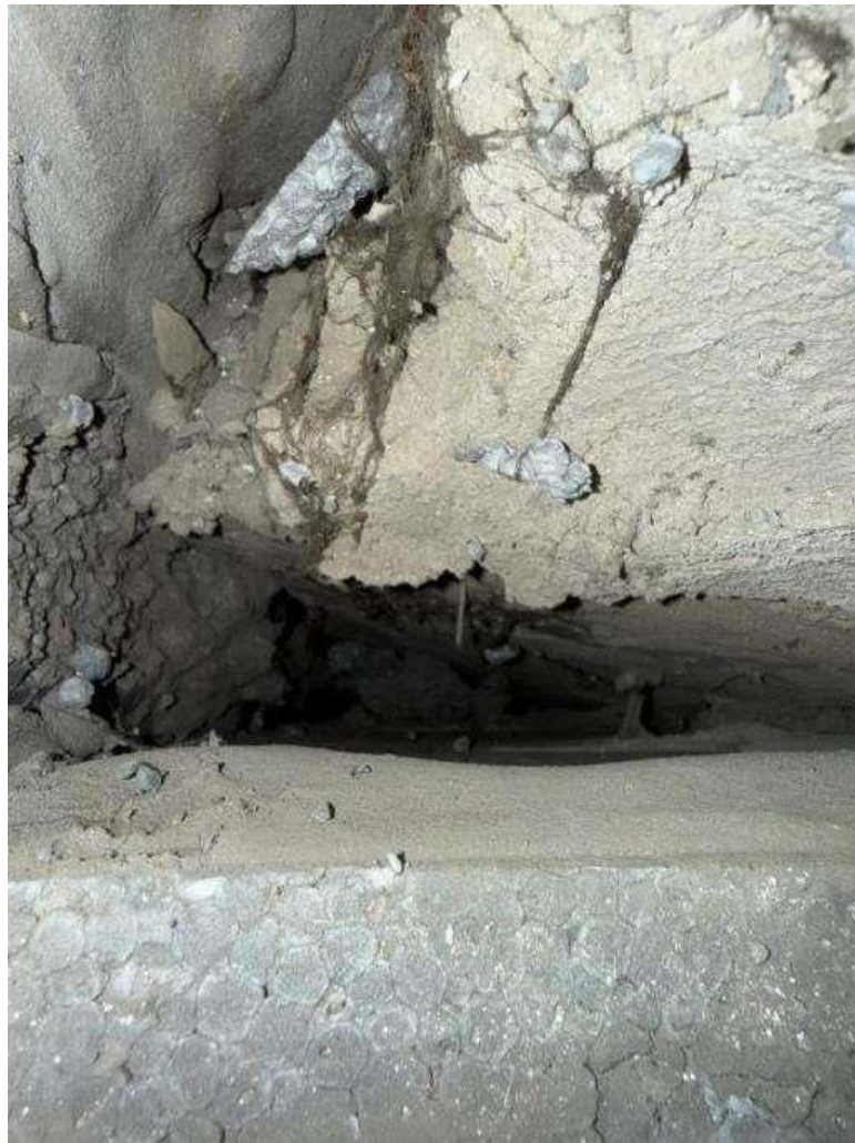
Figure 5.1.55. Gap up to 50 mm between the insulation and the wall
