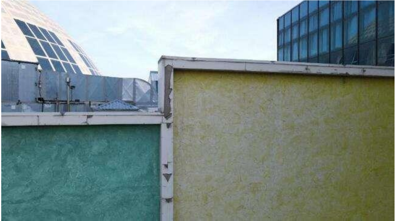
Figure 5.1.14. Damage to the finishing layer of imposts
