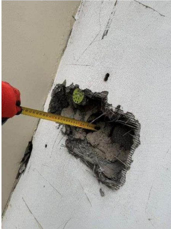
Figure 5.1.44. Exposure of the wall finishing layer
