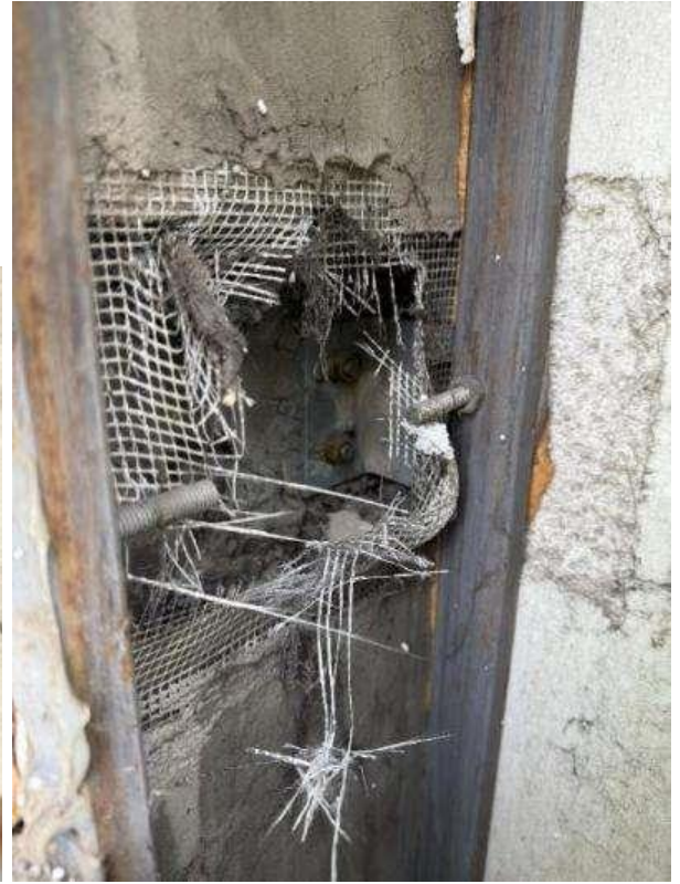
Figure 5.1.48. Fastening of the building impost frame to the wall
