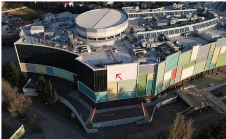
Figure 7.3 Recommended area for fencing in axes 5-6/A. Separation of insulation boards from the surface
