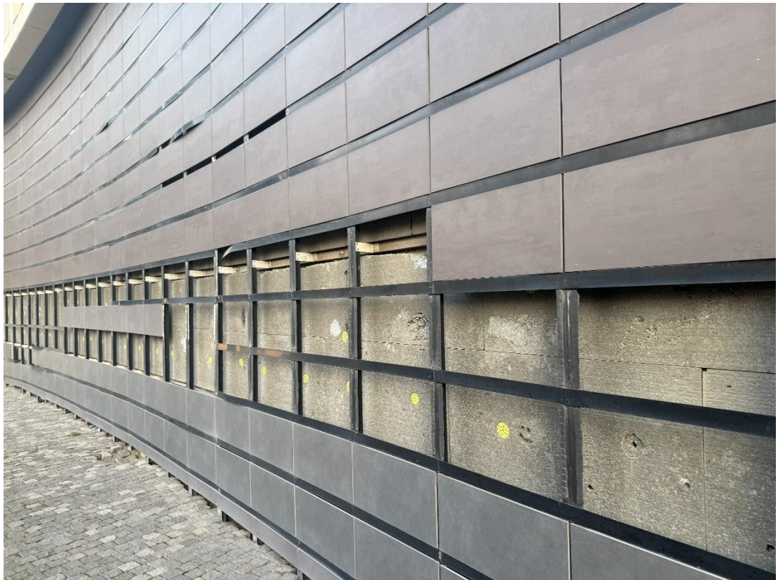
Figure 5.2.8. Detachment of slats and panels from frame posts. Enlarged joints between slabs
