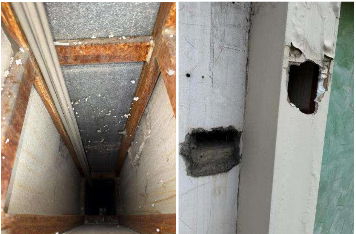
Figure 5.1.47. Corrosion of the building impost frame
