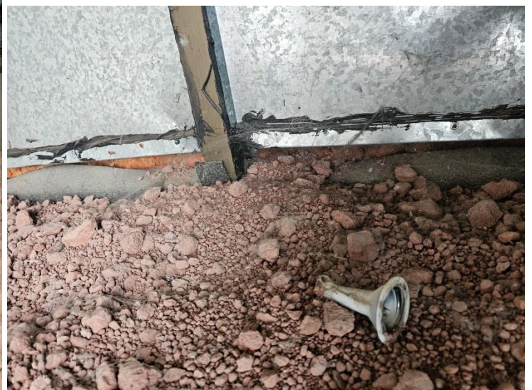
Figure 5.2.28. The ventilation grilles are currently not functional. These grilles are subject to leaks from precipitation (indirect defects). The inside is sealed with steel sheets and polyurethane sealant
