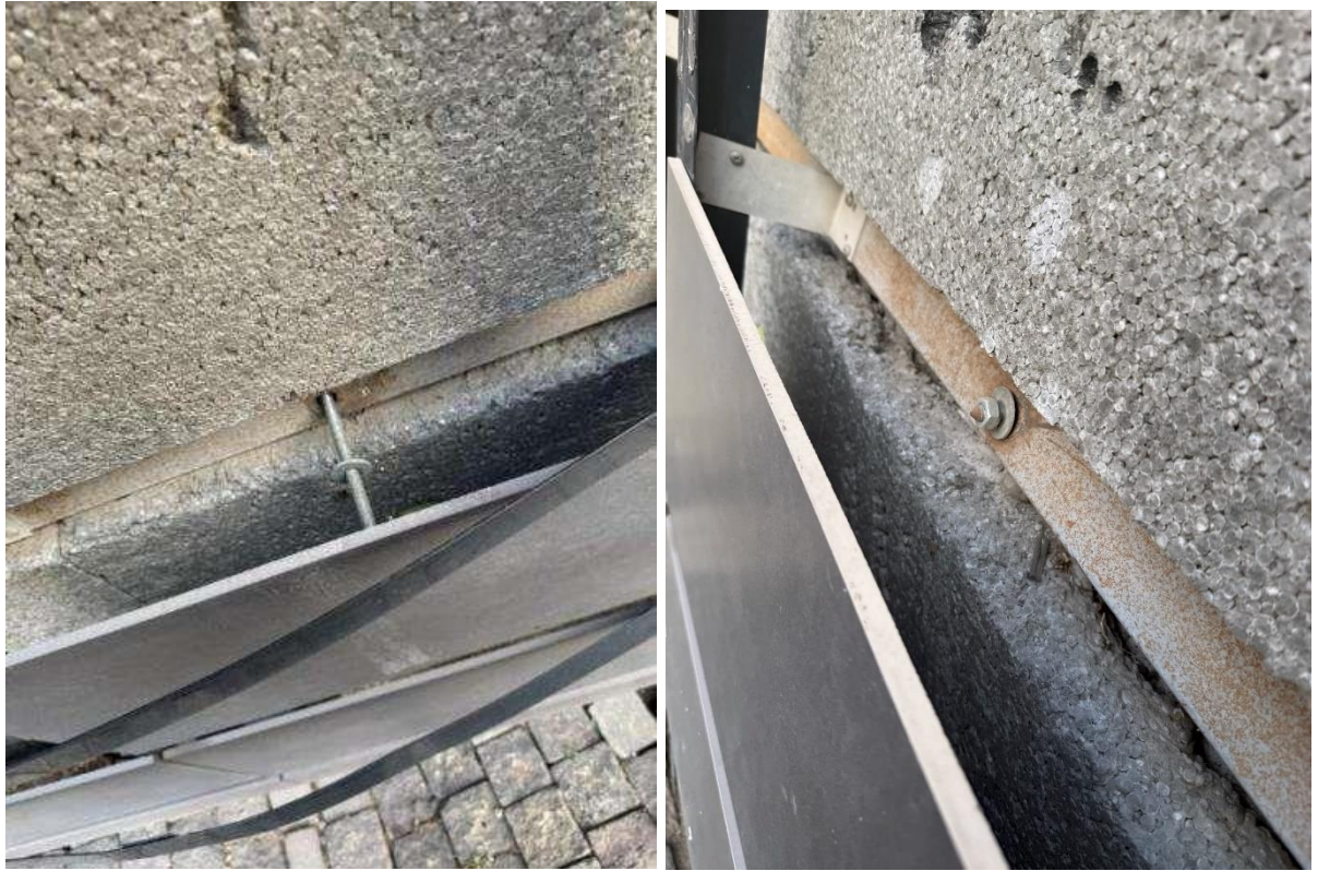
Figure 5.2.5. Failure to tighten the nut securing the frame to the wall
