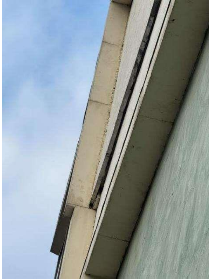
Figure 5.1.29. Lack of insulation layer adhesion along axis 5-6/A
