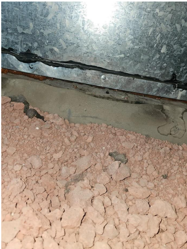
Figure 5.2.28. The ventilation grilles are currently not functional. These grilles are subject to leaks from precipitation (indirect defects). The inside is sealed with steel sheets and polyurethane sealant
