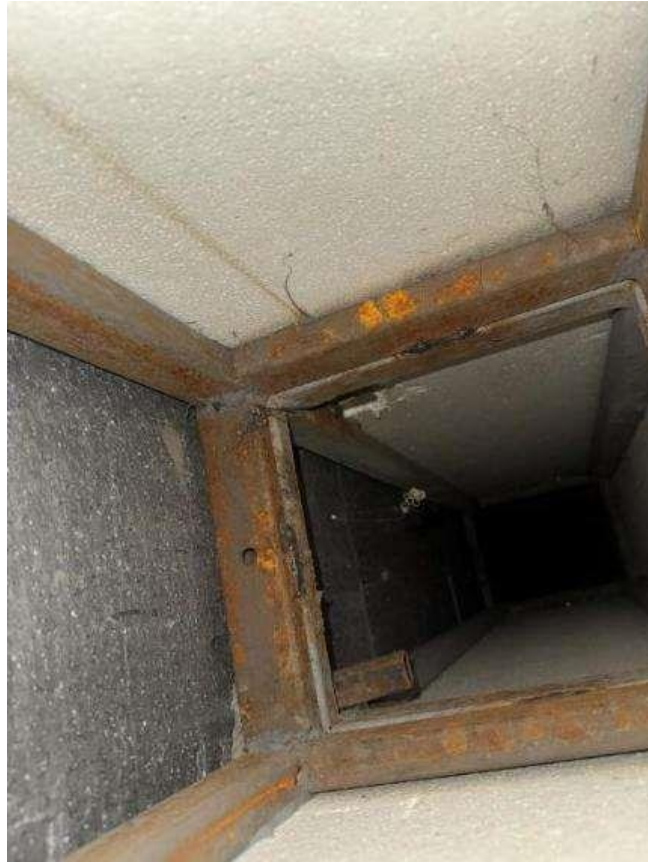
Figure 5.1.52. Corrosion of the impost frame
