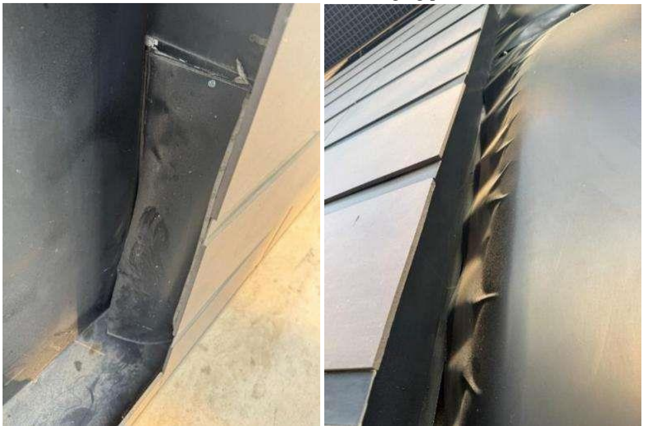
Figure 5.2.12. Destruction of the seam in the inscription "TBILISI MALL". Corrosion of the facade system frame
