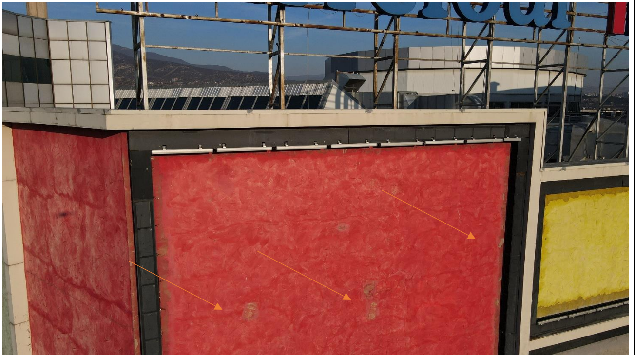
Figure 5.1.18. Space for a banner. Areas of facade damage
