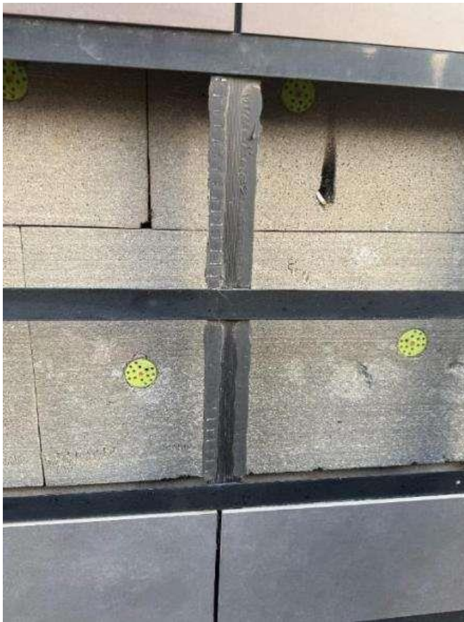
Figure 5.2.2. Fastenings of the insulation layer (insufficient). Increased gaps between slabs. Adhesive layer on the vertical fastening element of the ventilated facade
