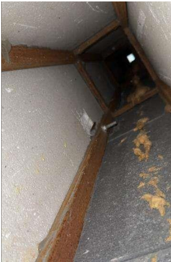
Figure 5.1.50. Fastening the building impost frame to the wall
