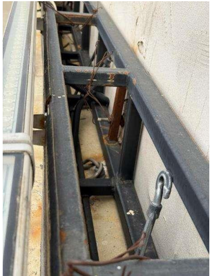
Figure 5.1.37. Fastening of the frame for placing banners. Lack of a clamping nut on the fastener
