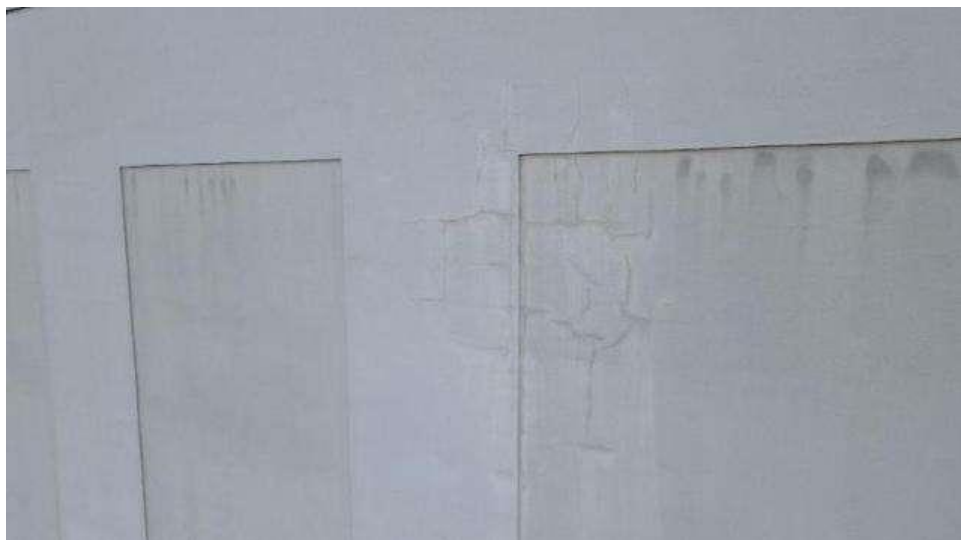
Figure 5.1.57. Cracks in the plaster layer of a lightweight insulation system
