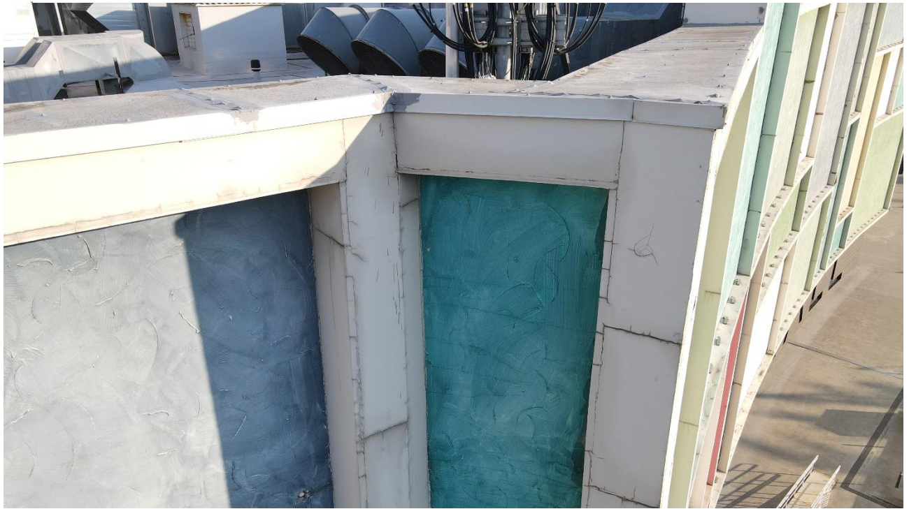
Figure 5.1.1 2. Cracks in the finishing layer of vertical imposts
