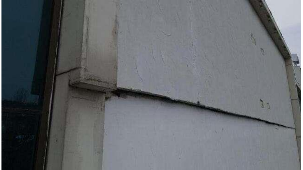
Figure 5.1.61. Crack on the facade of the building in axes 5-6/A. Delamination of the insulation layer.
