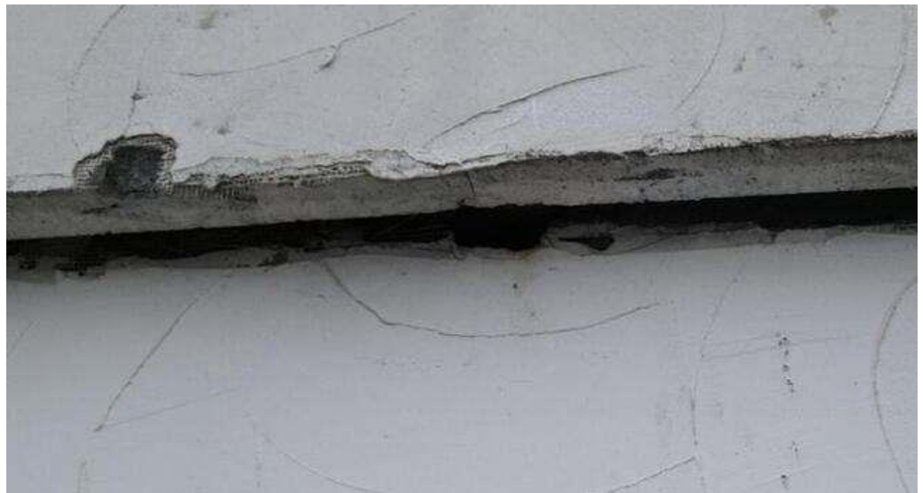
Figure 5.1.63. Crack on the building facade in axes 5-6/A. Delamination of the insulation layer.
