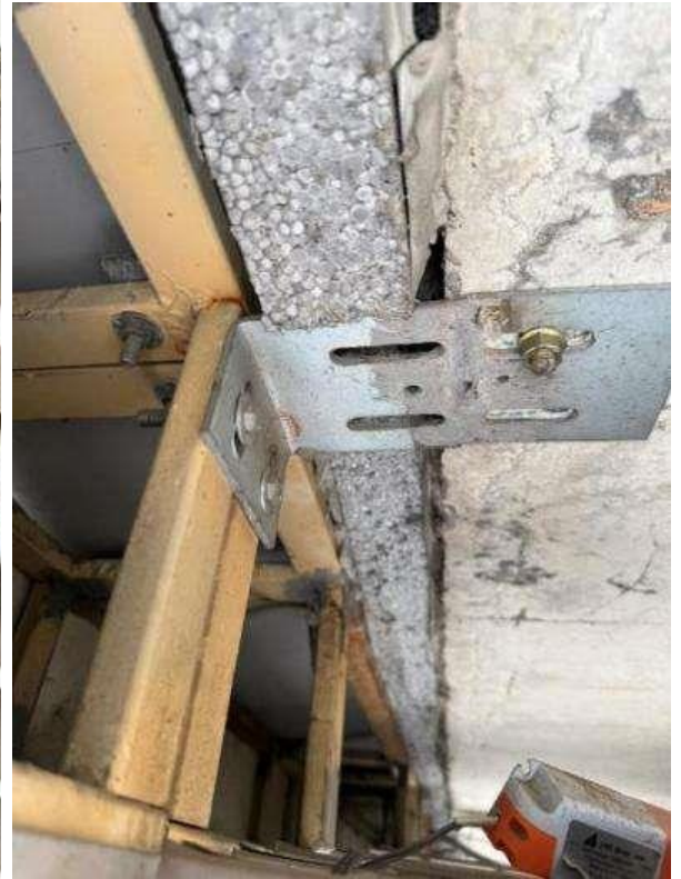
Figure 5.1.35. Fastening of the impost frame to the slab at elevation +6.000. Corrosion of frame elements. Lack of a support profile for the insulation. Non-continuous gluing of the insulation
