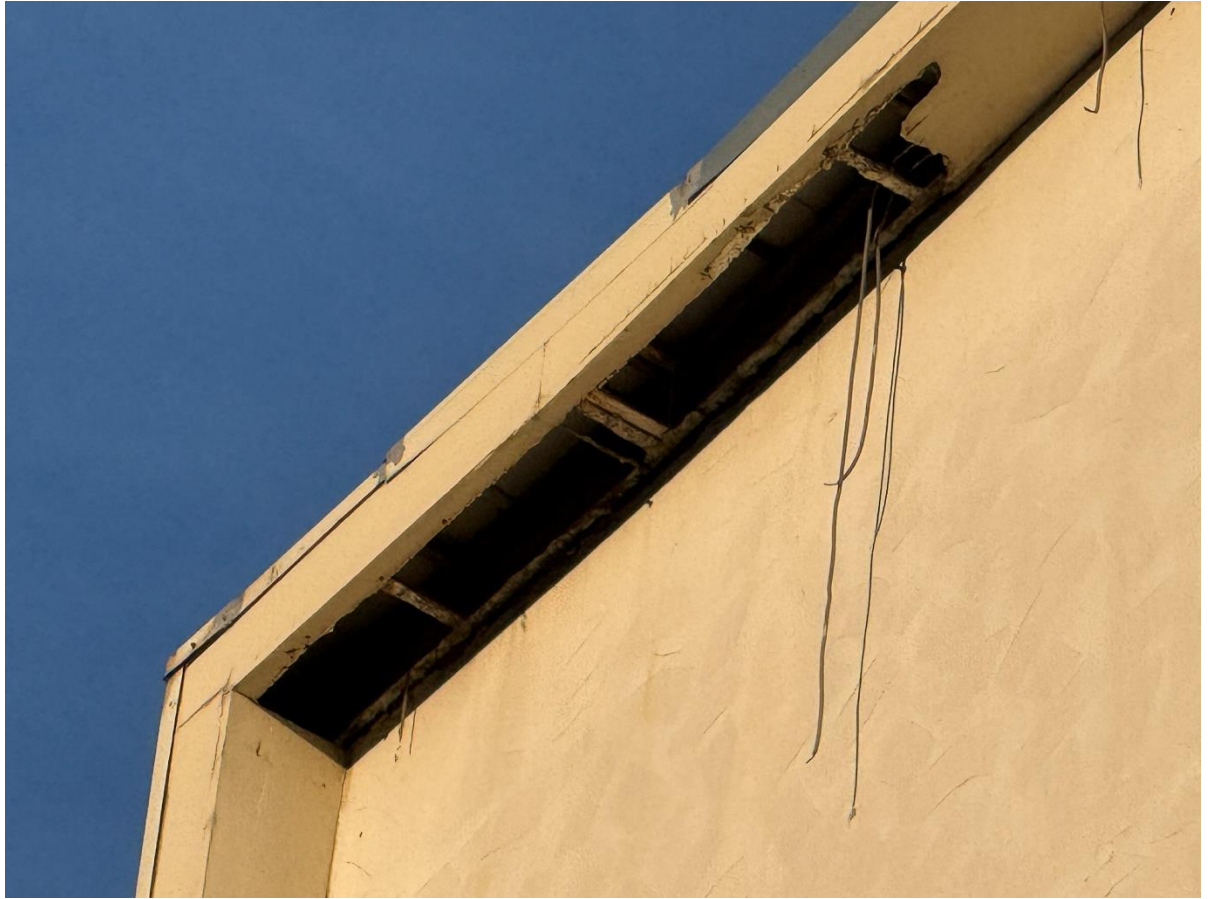
Figure 5.1.27. Destruction of the horizontal impost. Corrosion of the steel frame of the impost
