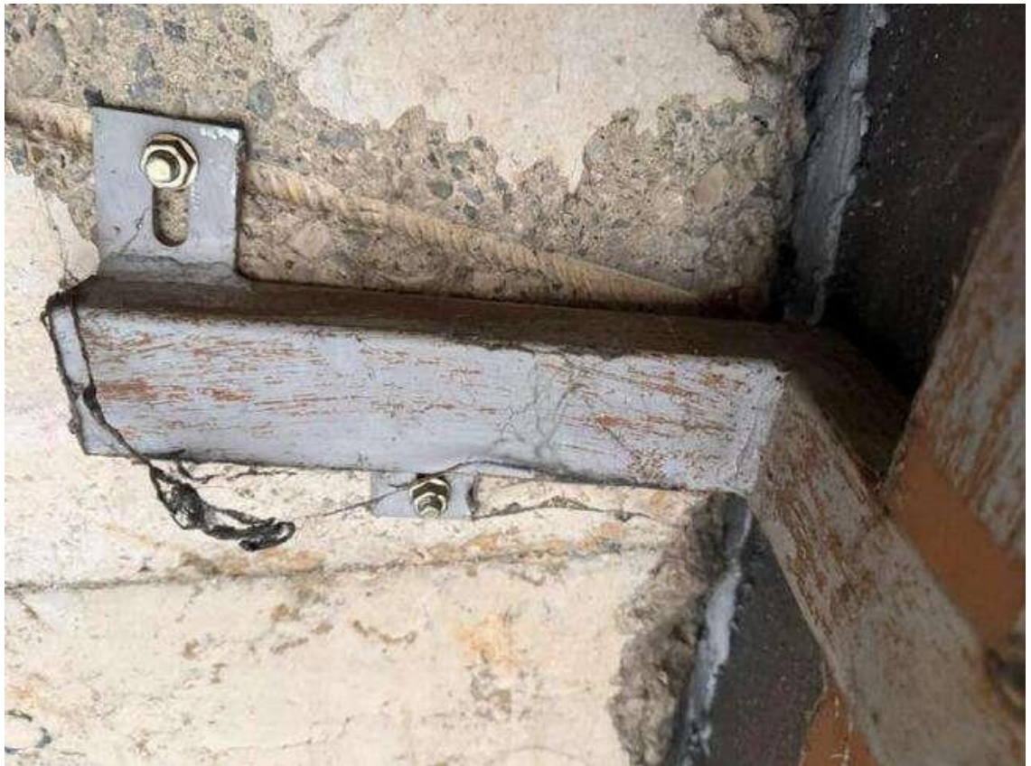
Figure 5.1.51. Fastening the building impost frame to the slab at elevation +6.000
