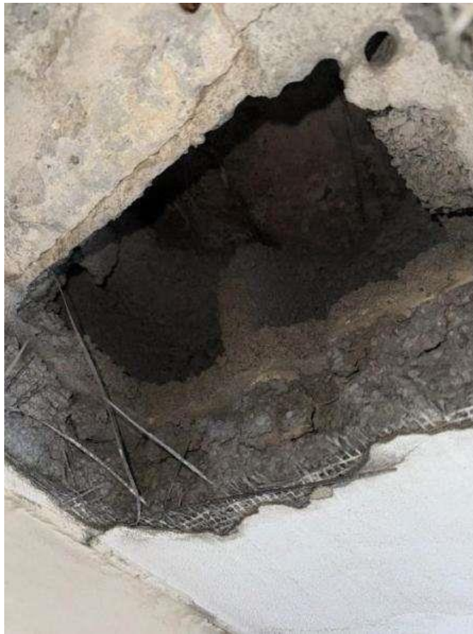
Figure 5.1.46. Aerated concrete block of the building wall
