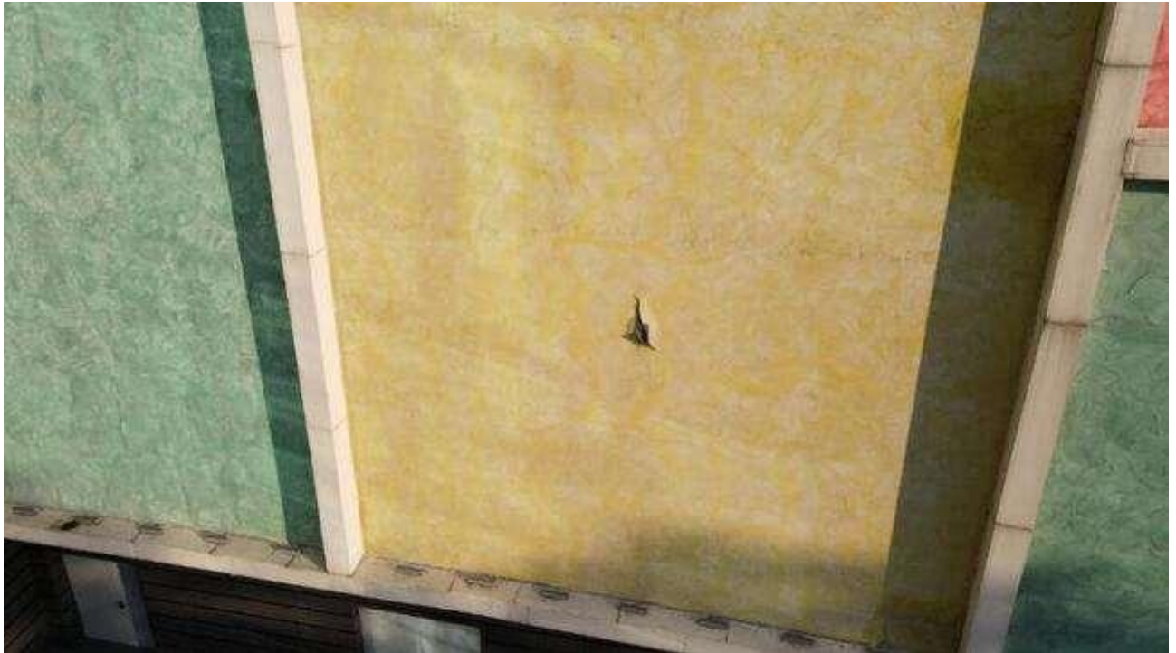
Figure 5.1.15. Localized damage to the PPS insulation layer
