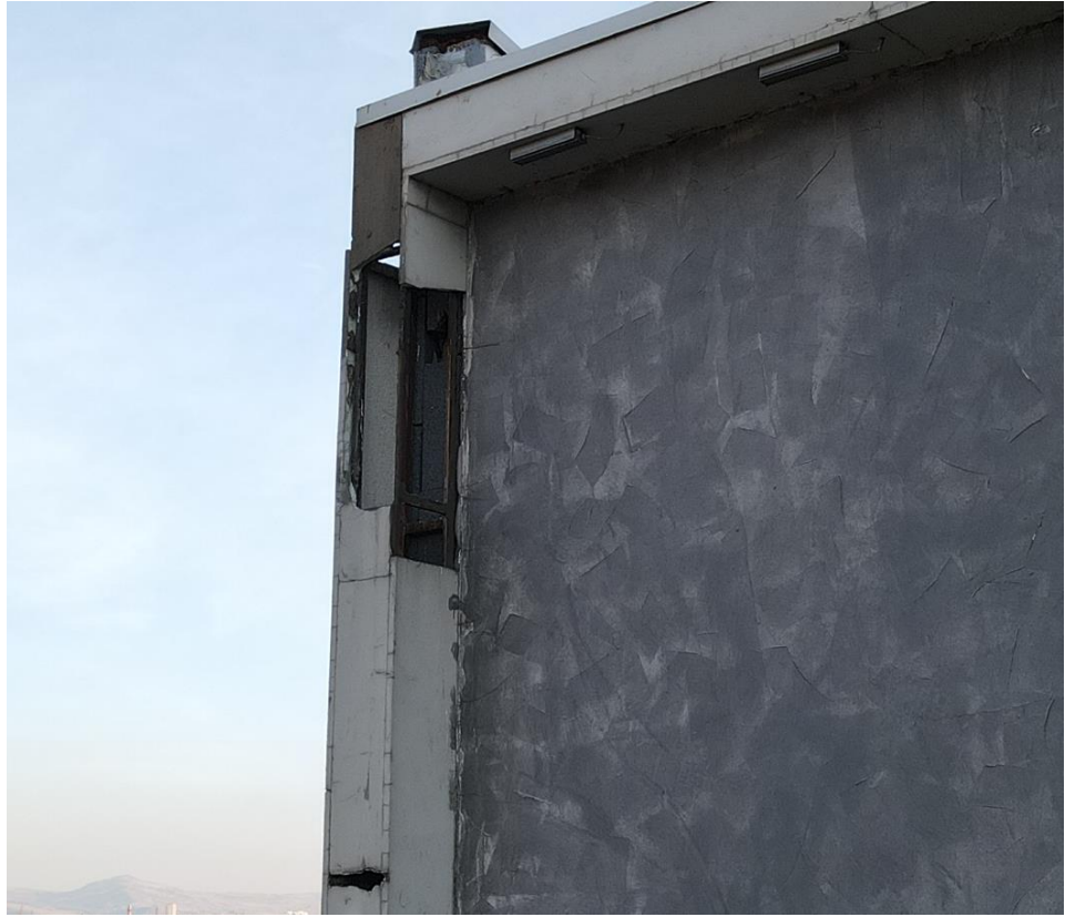
Figure 5.1.25. Destruction of vertical impost. Corrosion of steel impost frame along axis 6/C
