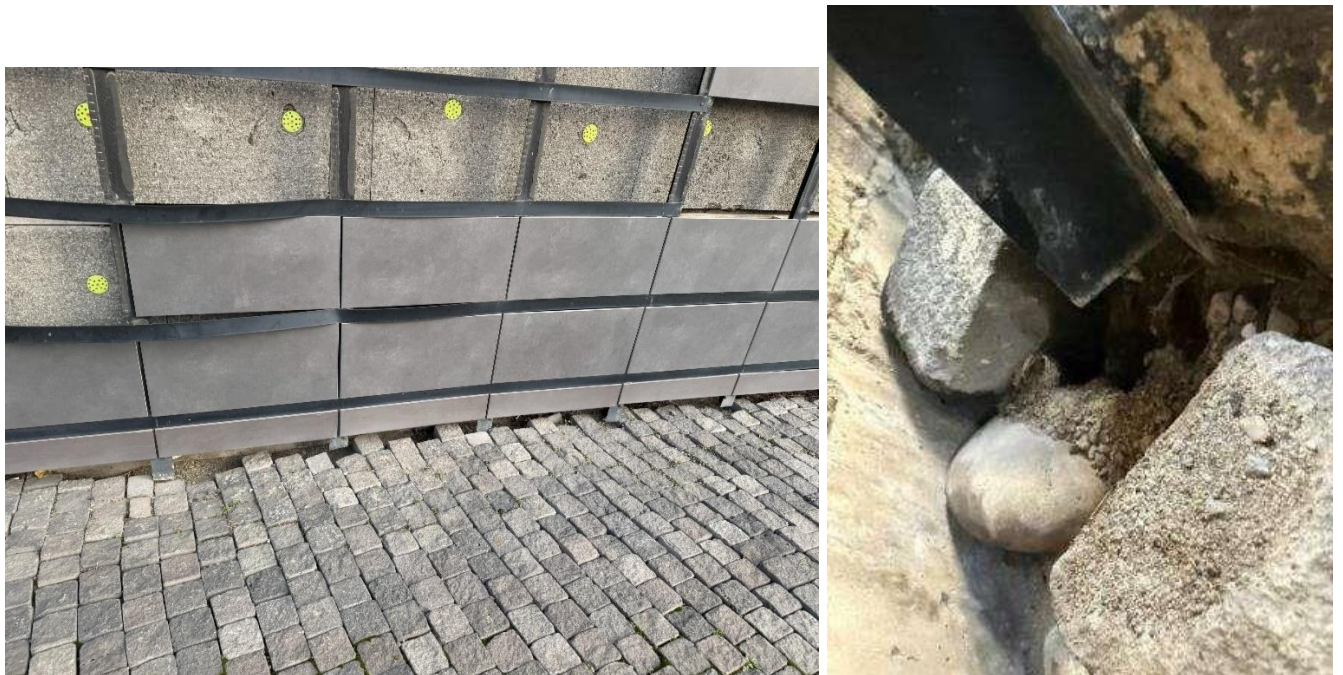
Figure 5.2.4. Delamination of slats and panels from the frame uprights
