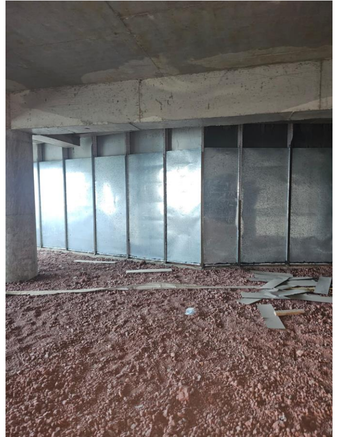
Figure 5.2.27. The ventilation grilles are currently not functional. These grilles are subject to leaks from precipitation (indirect defects). The inside is sealed with steel sheets and polyurethane sealant.
