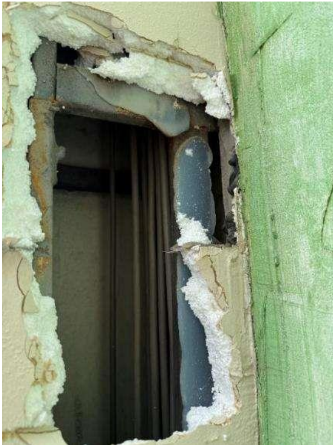
Figure 5.1.32. Opening of the vertical impost. Areas of adhesive bonding (non-continuous). This method of fastening is not standardized; similar solutions must also be mechanically fastened due to the small contact area
