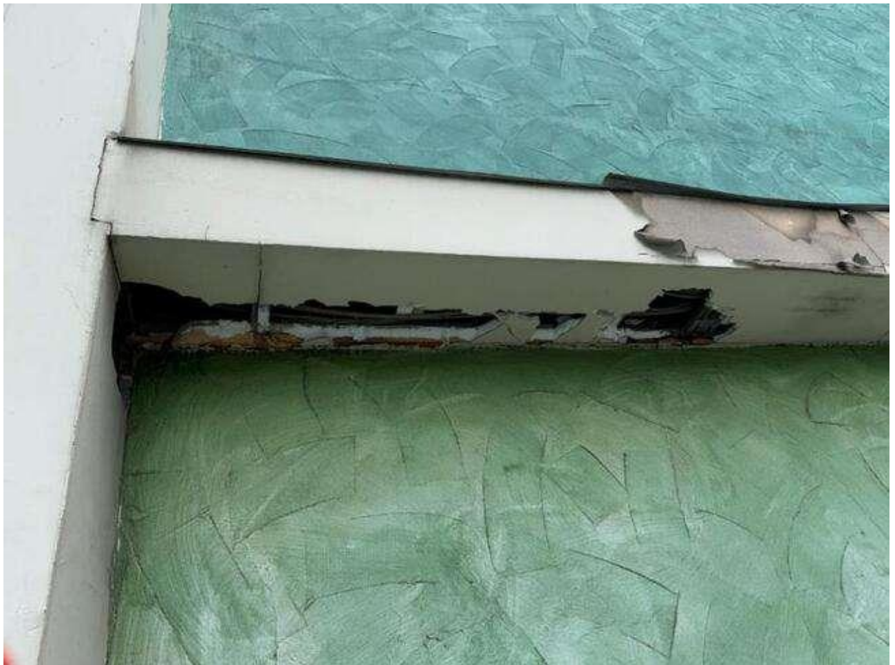
Figure 5.1.42. Opening the finishing layer of the horizontal impost
