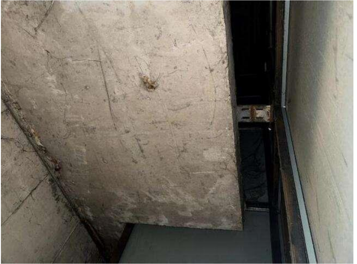
Figure 5.2.21. Corrosion of the frame of the suspended aluminum facade panels
