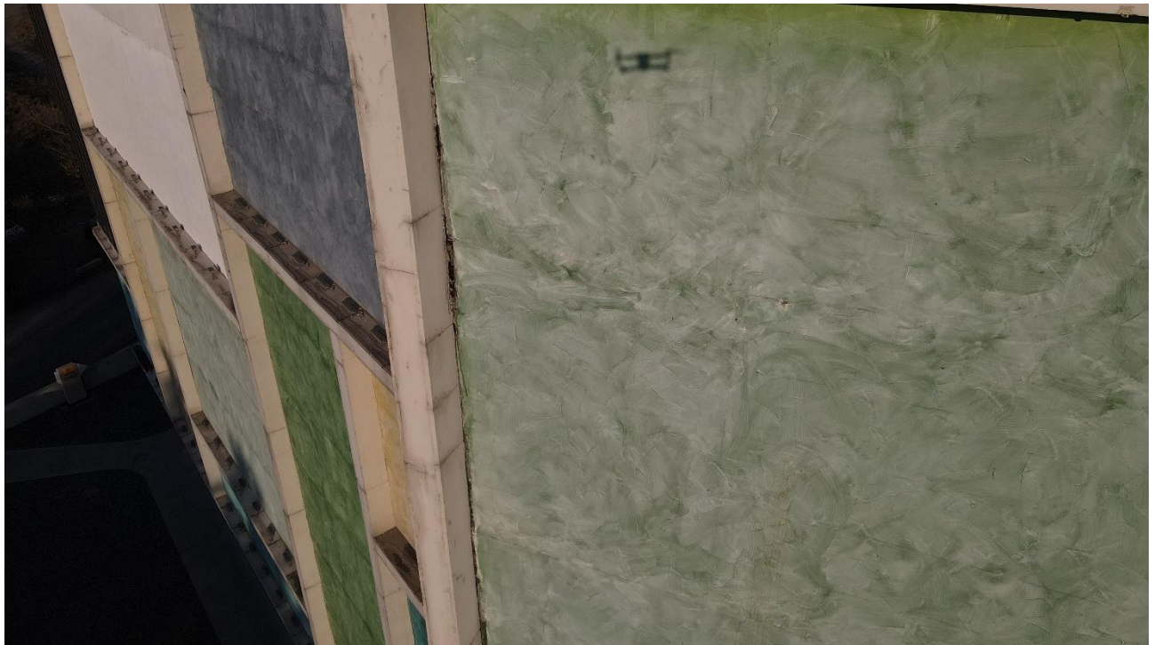
Figure 5.1.12. Damage to the junction between wall insulation and vertical jamb
