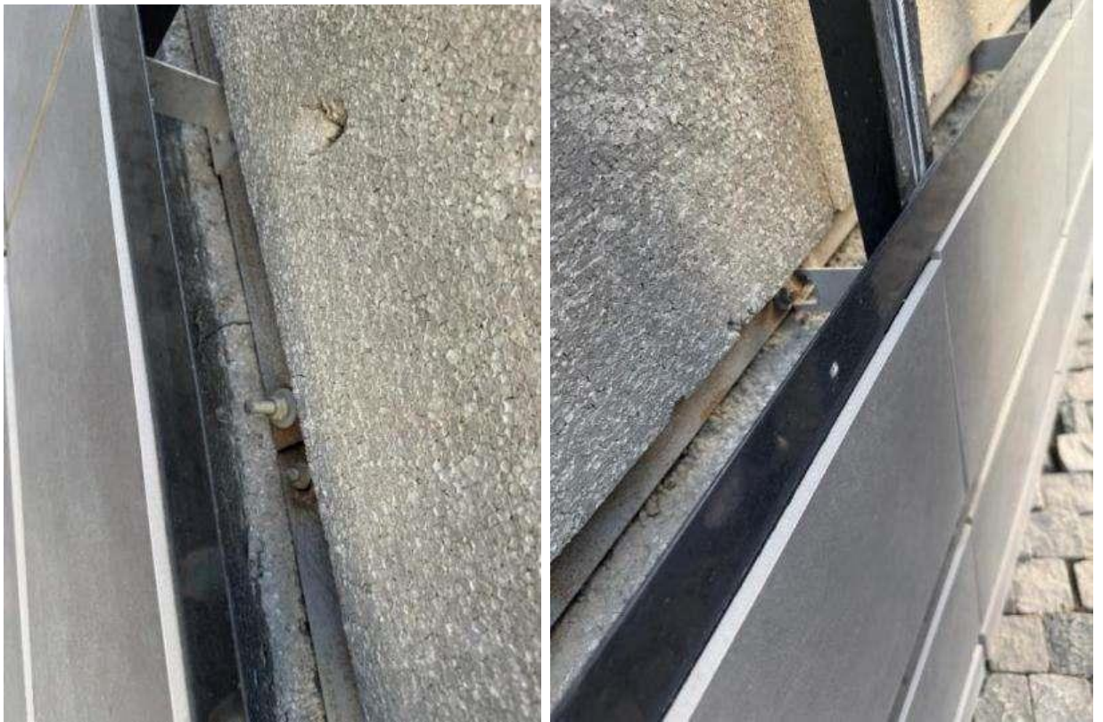
Figure 5.2.3. Fastening of the facade frame to the wall
