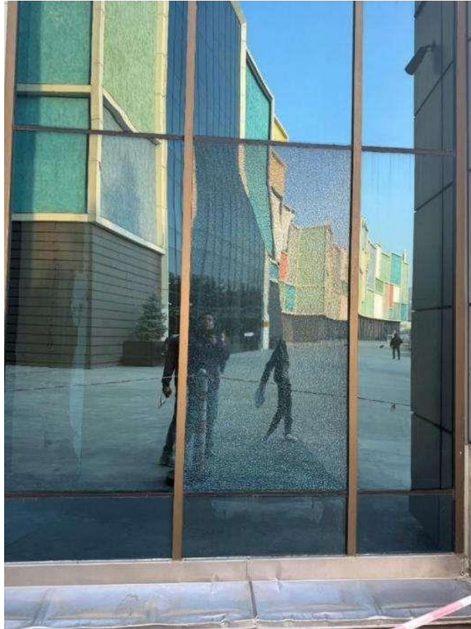
Figure 5.2.15. Broken stained glass window in axes 3/A
