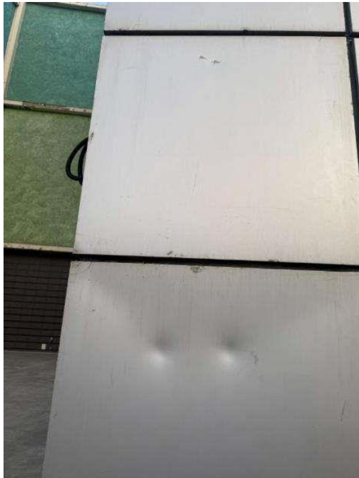
Figure 5.2.16. Mechanical damage (dents) on aluminum panels in axes 2-3/A'
