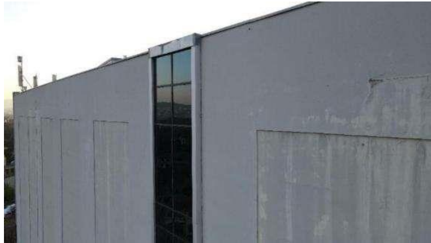
Figure 5.1.59. Peeling of the finishing layer. Cracks in the plaster layer of the facade in axes 1-6/C
