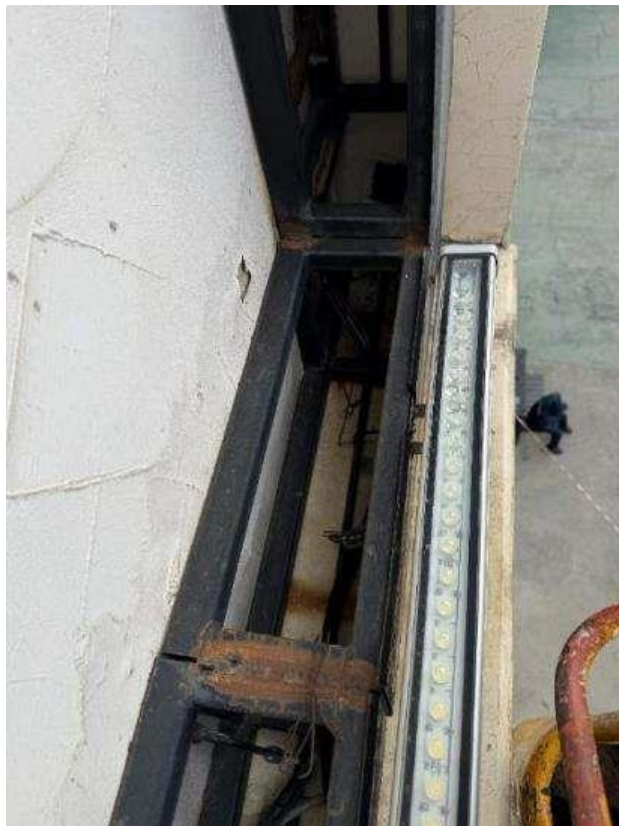
Figure 5.1.36. Frame for placing banners. Talpers in the frame structure. Corrosion of welded joints
