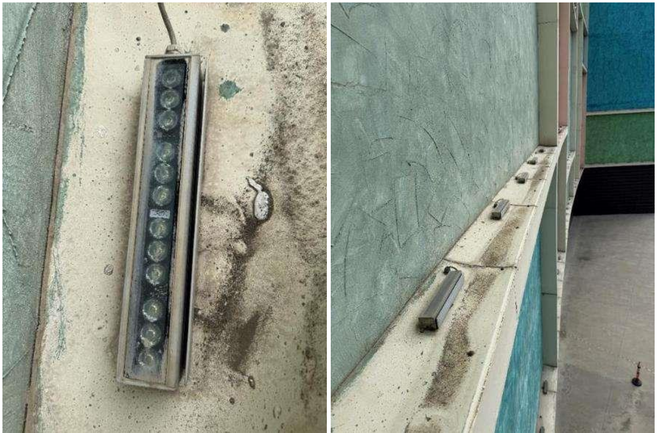
Figure 5.1.34. Facade lighting in the design of horizontal imposts
