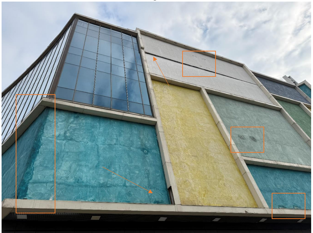
Figure 5.1.28. Areas of facade damage. Unsatisfactory facade construction (insulation delamination). Damage to the impost.
