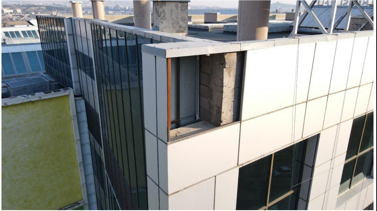
Figure 5.2.25. Absence of aluminum panels on the facade
