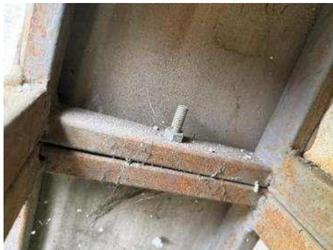
Figure 5.1.49. Fastening the frame of the building impost to the wall. Connecting the frame elements to each other
