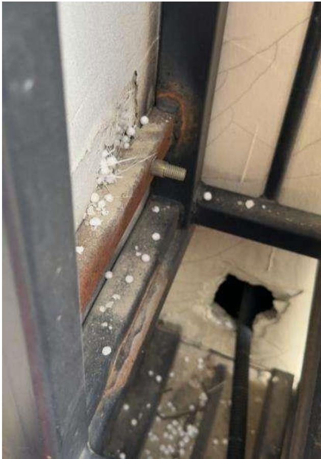
Figure 5.1.37. Fastening of the frame for placing banners. Lack of a clamping nut on the fastener
