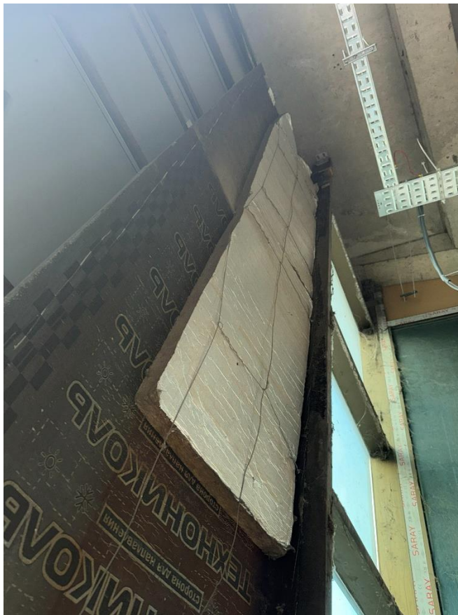
Figure 5.2.18. Insulation structure of this part of the facade
