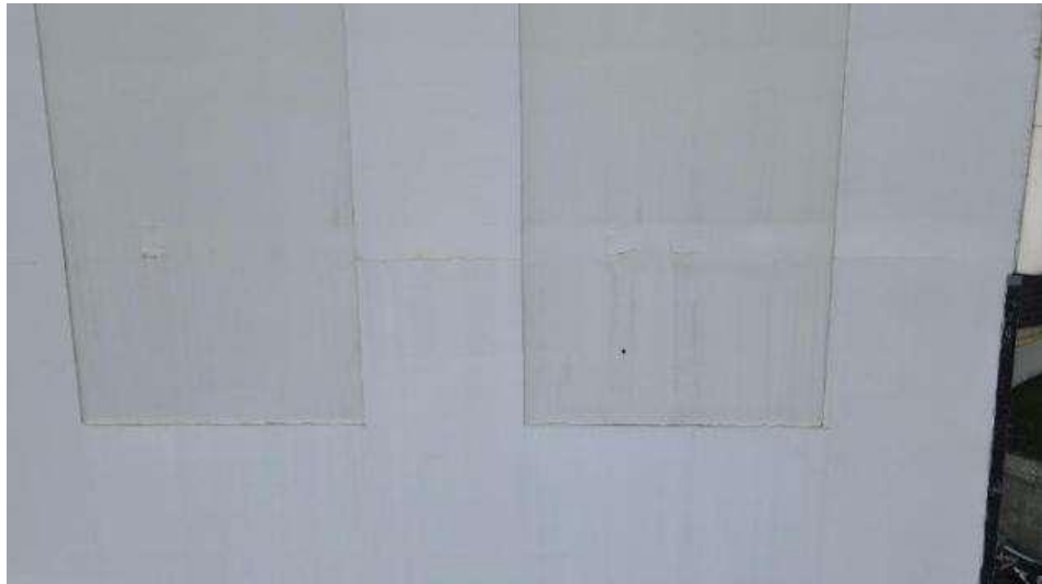
Figure 5.1.56. Cracks in the plaster layer of the lightweight insulation system in axes 1-6/C
