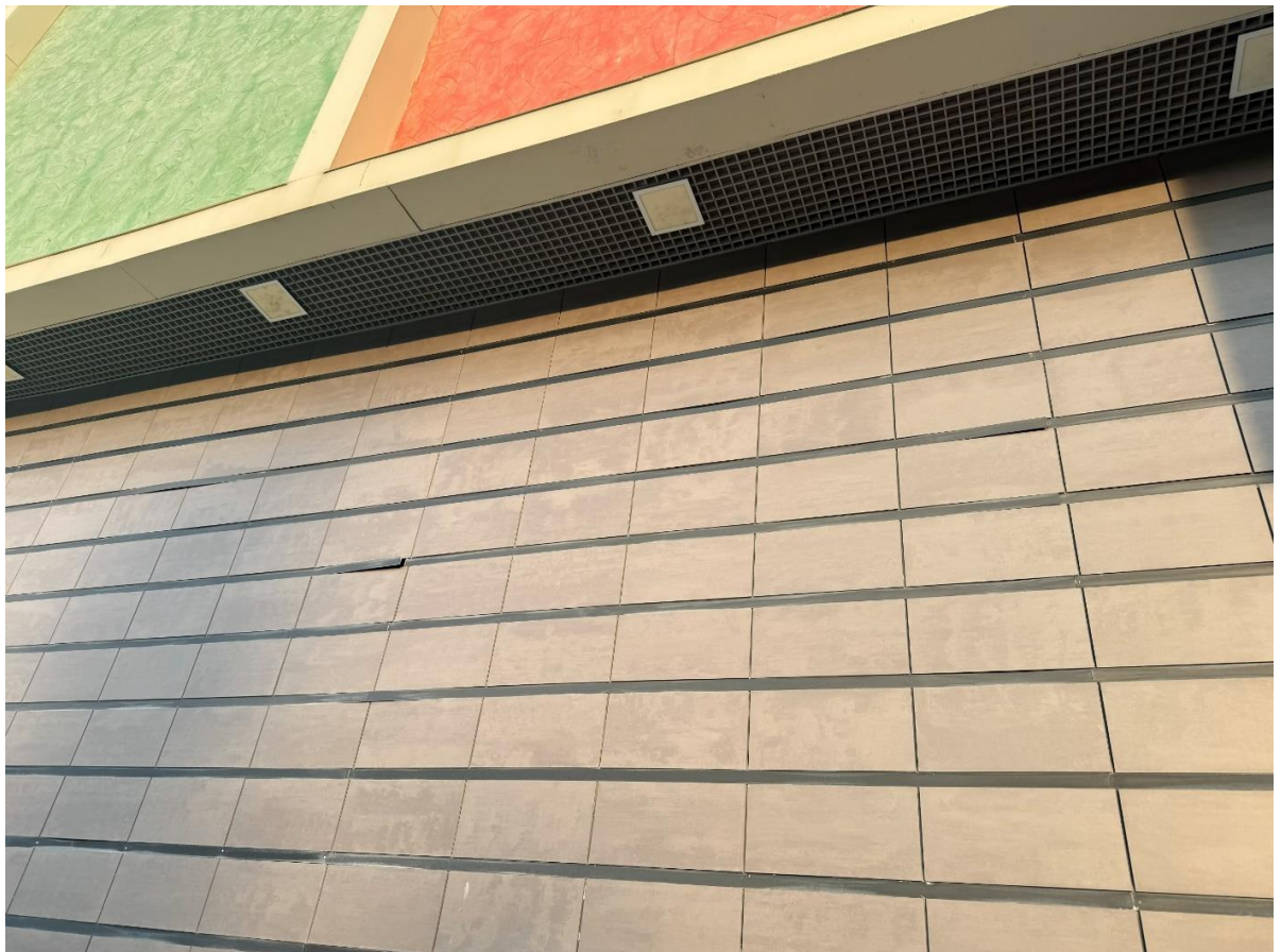
Figure 5.2.10. Delamination of lamellas and panels from frame posts
