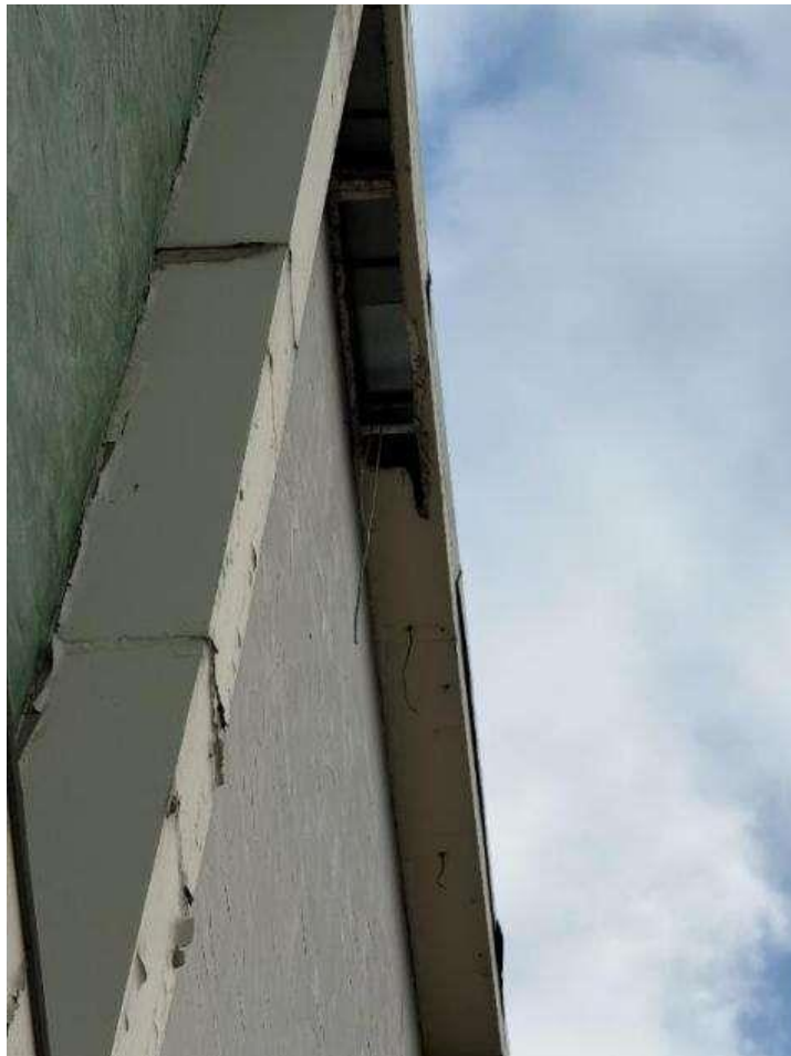
Figure 5.1.45. Destruction of the horizontal impot. Corrosion of the steel frame
