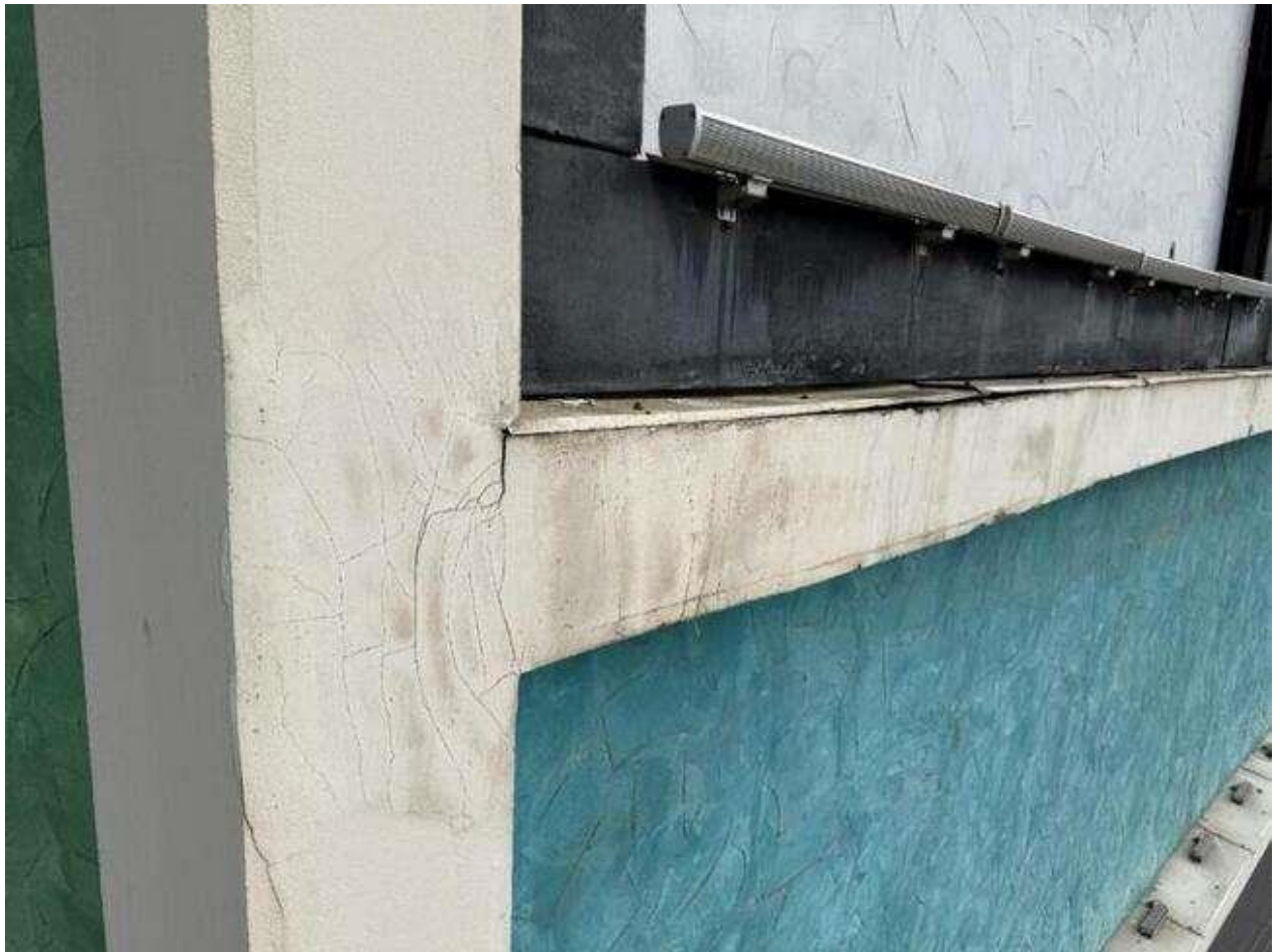
Figure 5.1.39. Cracks in the finishing layer of the horizontal impost
