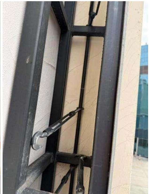
Figure 5.1.36. Frame for placing banners. Talpers in the frame structure. Corrosion of welded joints
