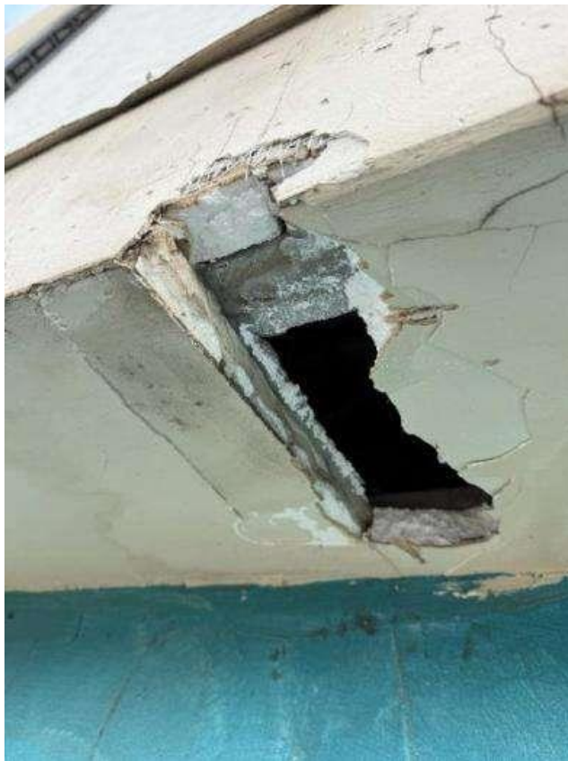
Figure 5.1.38. Opening of the horizontal impost. Areas of surface corrosion
