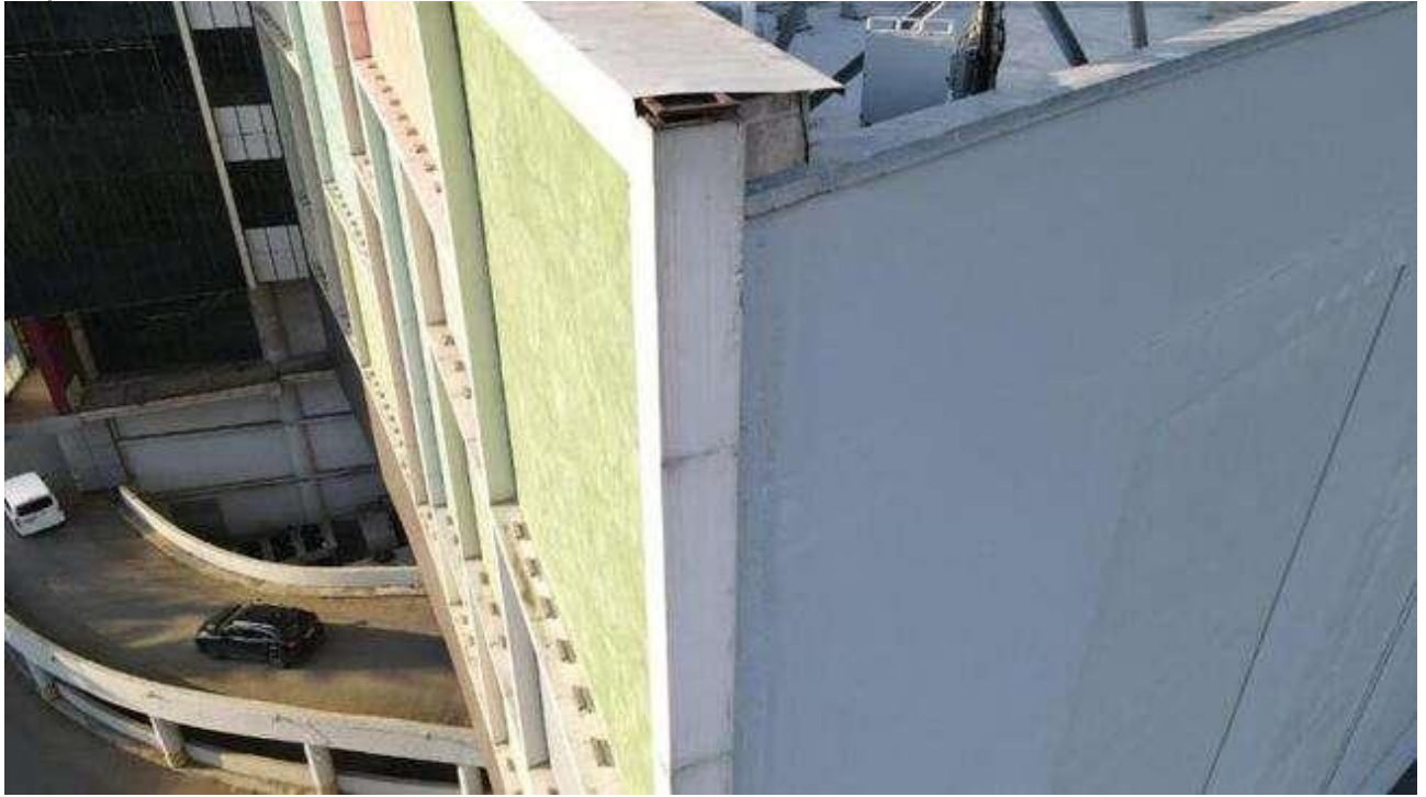
Figure 5.1.24. Facade junction along axis 1/C. Insufficient parapet overhang
