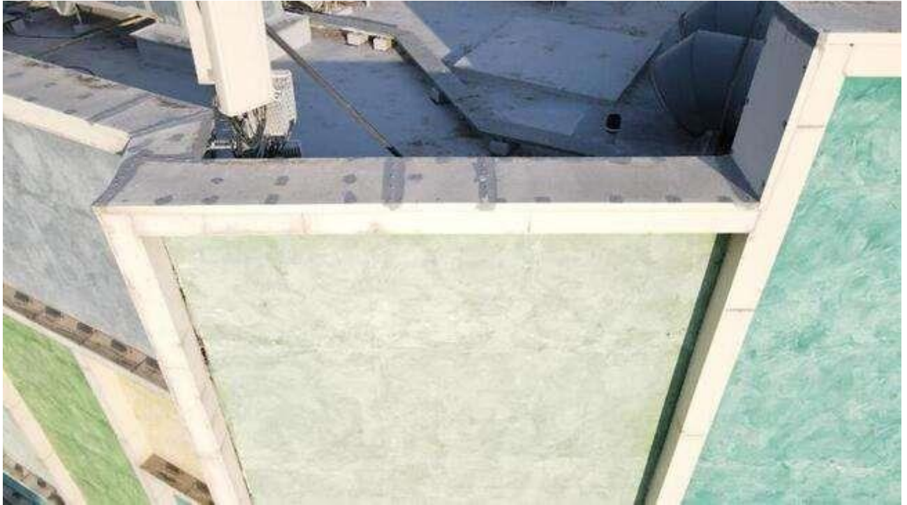
Figure 5.1.11. Drip molding along the upper edge of the facade. The joints of the drip molding are treated with sealant
