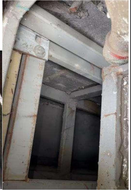
Figure 5.1.31. Connection of the vertical and horizontal frames of the facade impost. Surface corrosion
