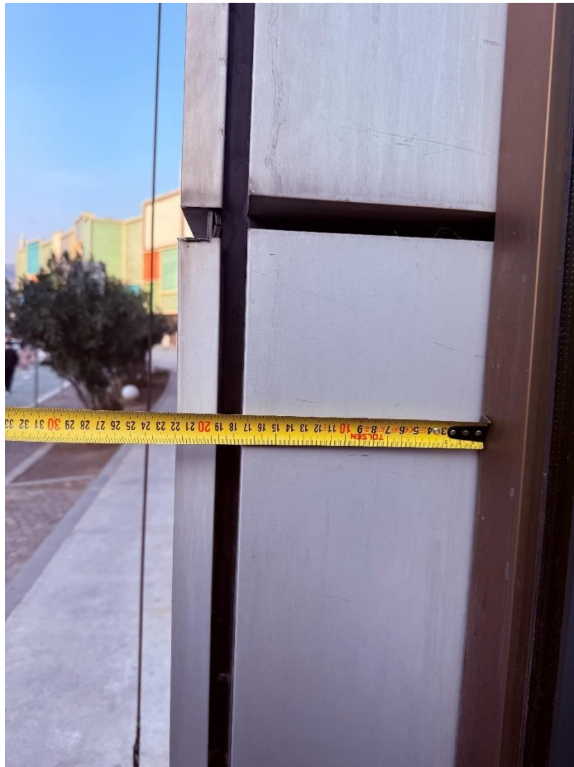
Figure 5.2.19. Seams of the facade with aluminum panels
