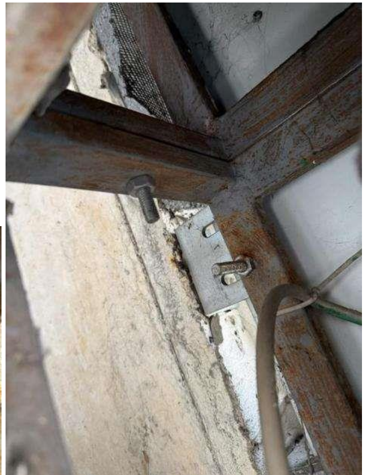
Figure 5.1.49. Fastening the frame of the building impost to the wall. Connecting the frame elements to each other
