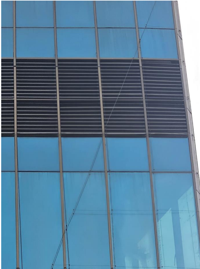
Figure 5.2.26. Ventilation grilles on the curtain wall in axes 1-3/A-C
