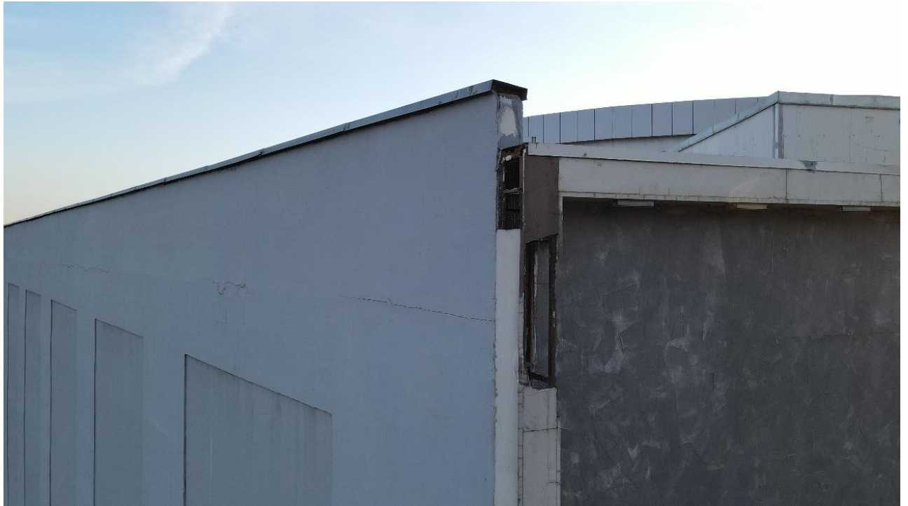
Figure 5.1.25. Facade junction along axis 6/C. Destruction of vertical impost
