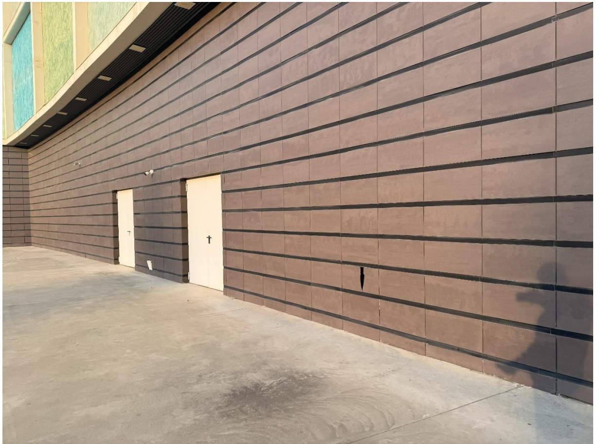
Figure 5.2.11. Delamination of battens and panels from frame studs with sealant. Cracks and destruction of hanging panels
