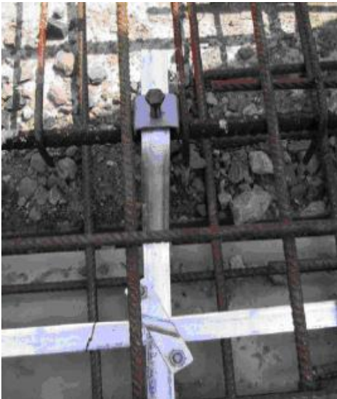
Photo 5: Connection example to rebar
