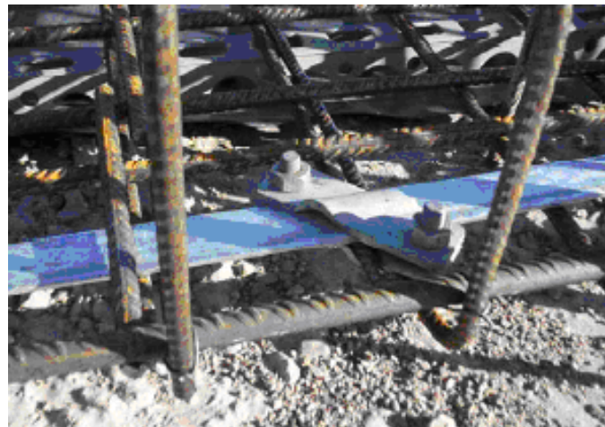
Photo 6: Connection example to rebar
