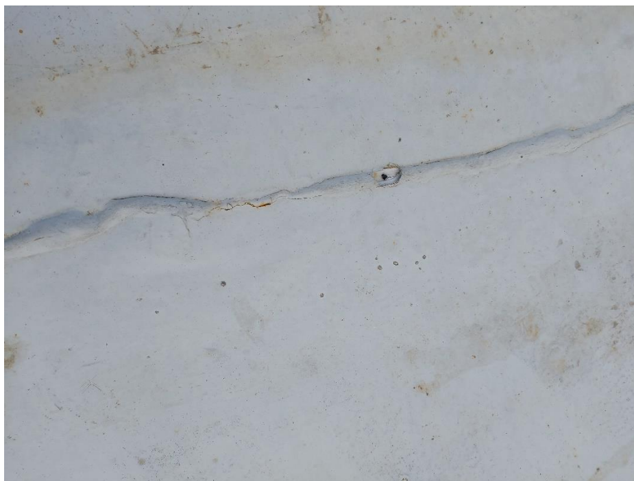
Existing waterproofing typical damages
