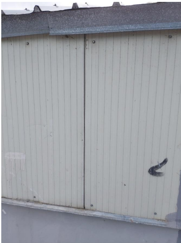
Skylight sandwich panels and seams
