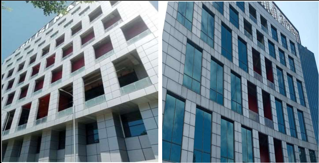
Aluminum Composite Panel Façade with Glass Handrails And Glass Façade
