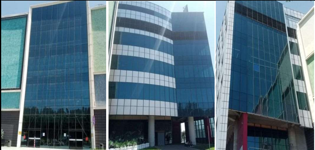
Glass Façade (front side)
